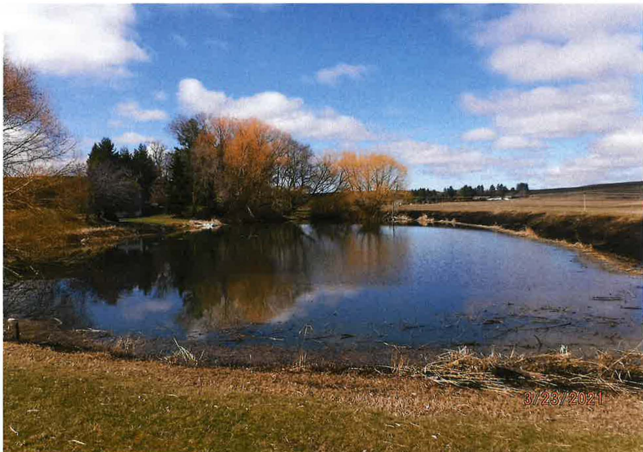
POU – IRRIGATION STORAGE & FIRE PROTECTION STORAGE
