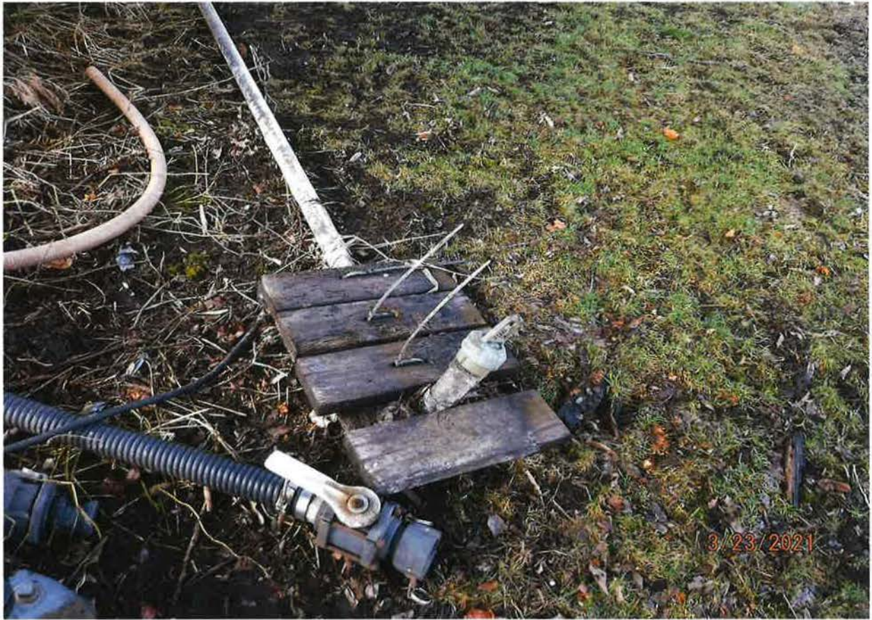
IRRIGATION FROM STORAGE – 30 FOOT FLOATING INTAKE PIPE TO PUMP
