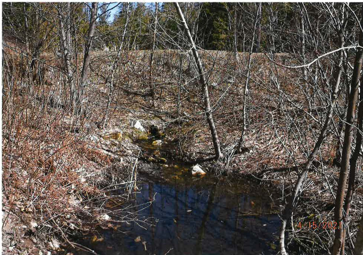
OVERFLOW DISCHARGE PIPE BELOW DAM
