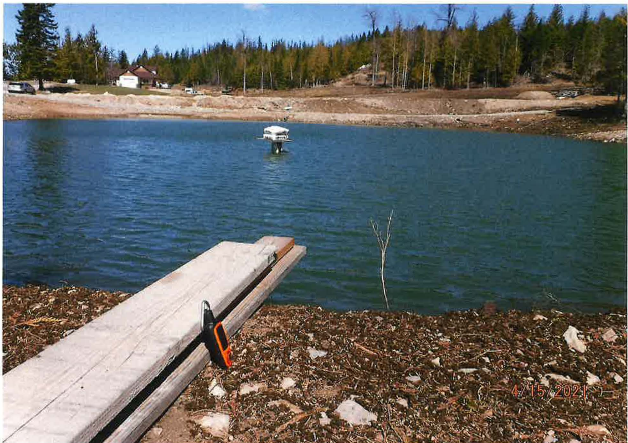
POD – EARTHEN DAM
