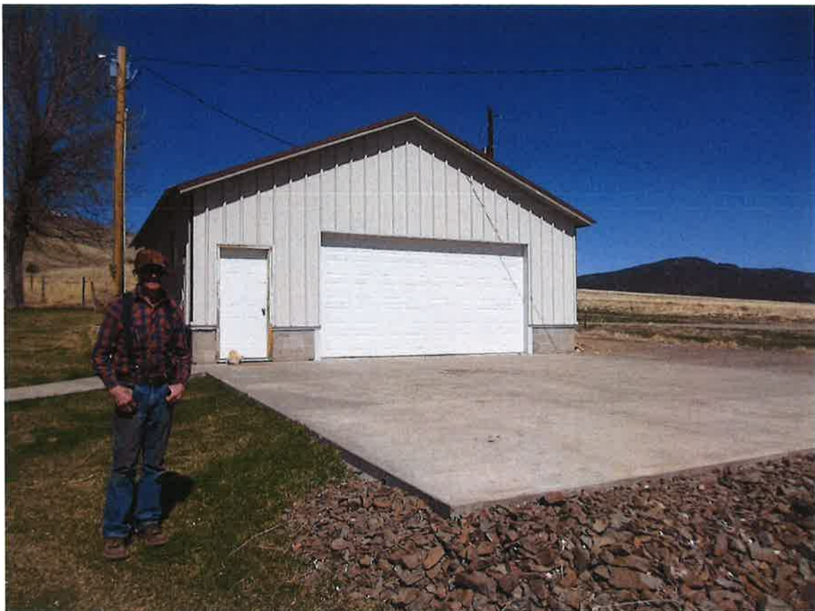
Place of Use – Heating - Garage and Heated Slab
