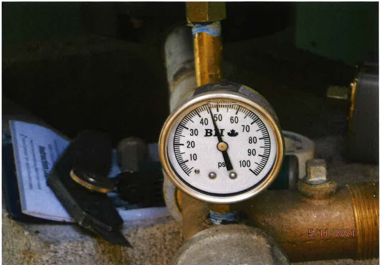
45 PSI SYSTEM OPERATING PRESSURE
