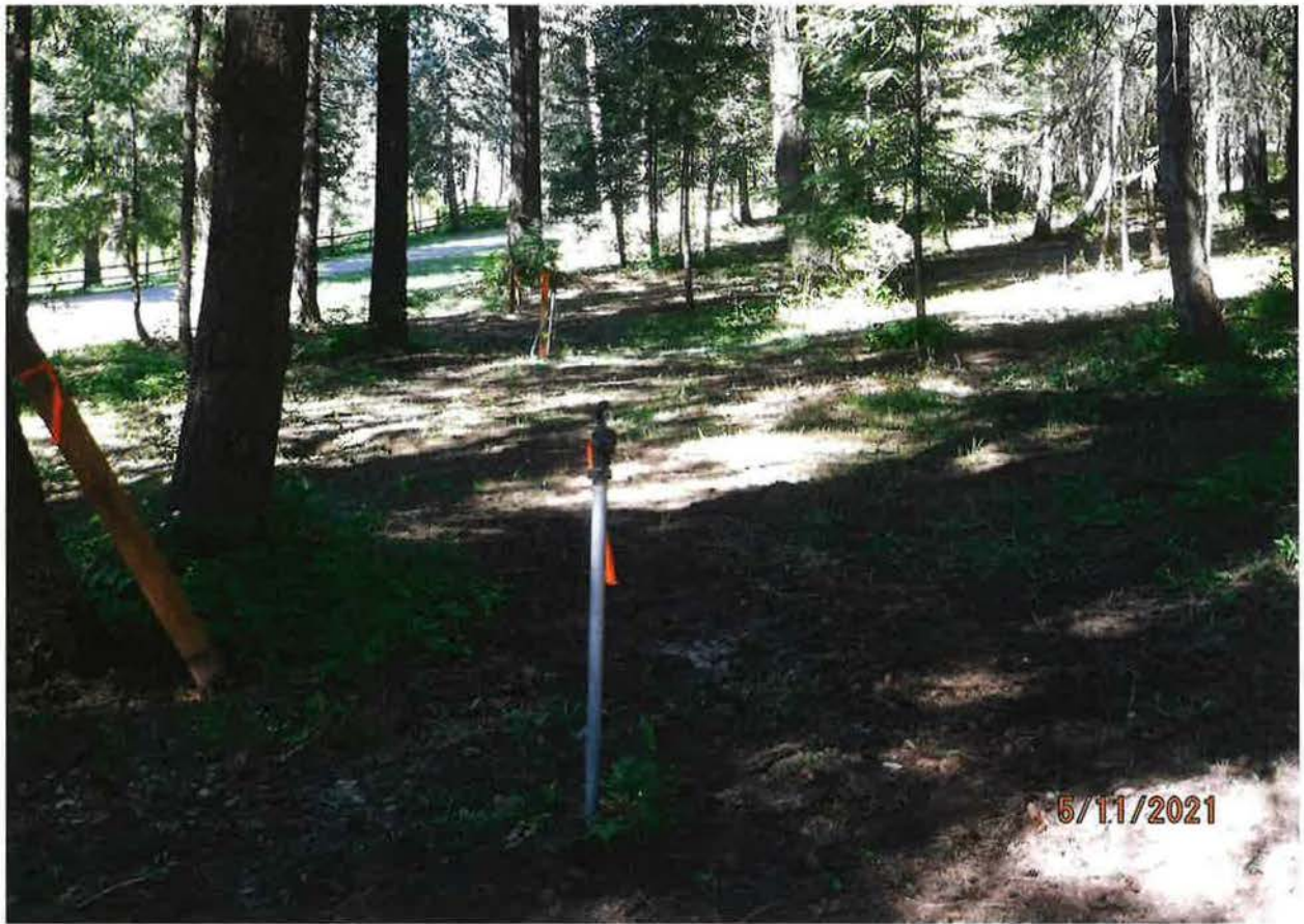
IRRIGATION POU – FROST FREE HYDRANTS AT INTERVALS UP HILL TO MAIN ROAD
