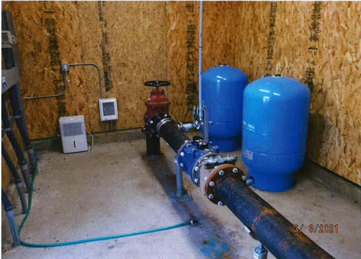
WATER SYSTEM DIVERTING WORKS WITH PRESSURE TANKS
