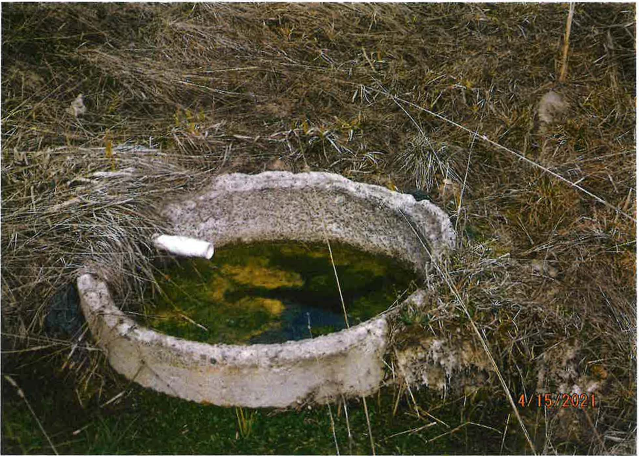
POD – SPRING SOURCE – SEEPS FROM SIDE HILL FILLING CONCRETE CISTERN
