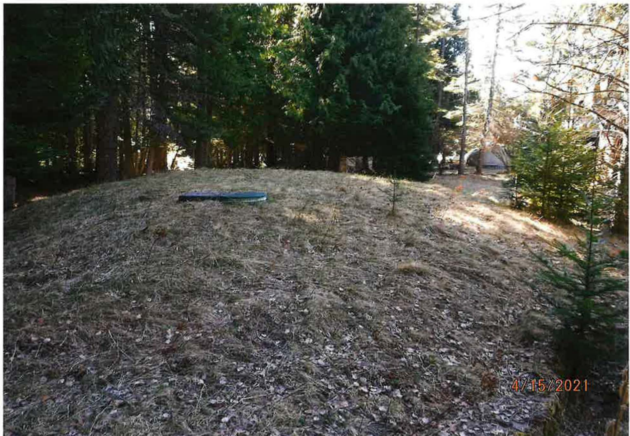
10,000 GAL STORAGE RESERVOIR
