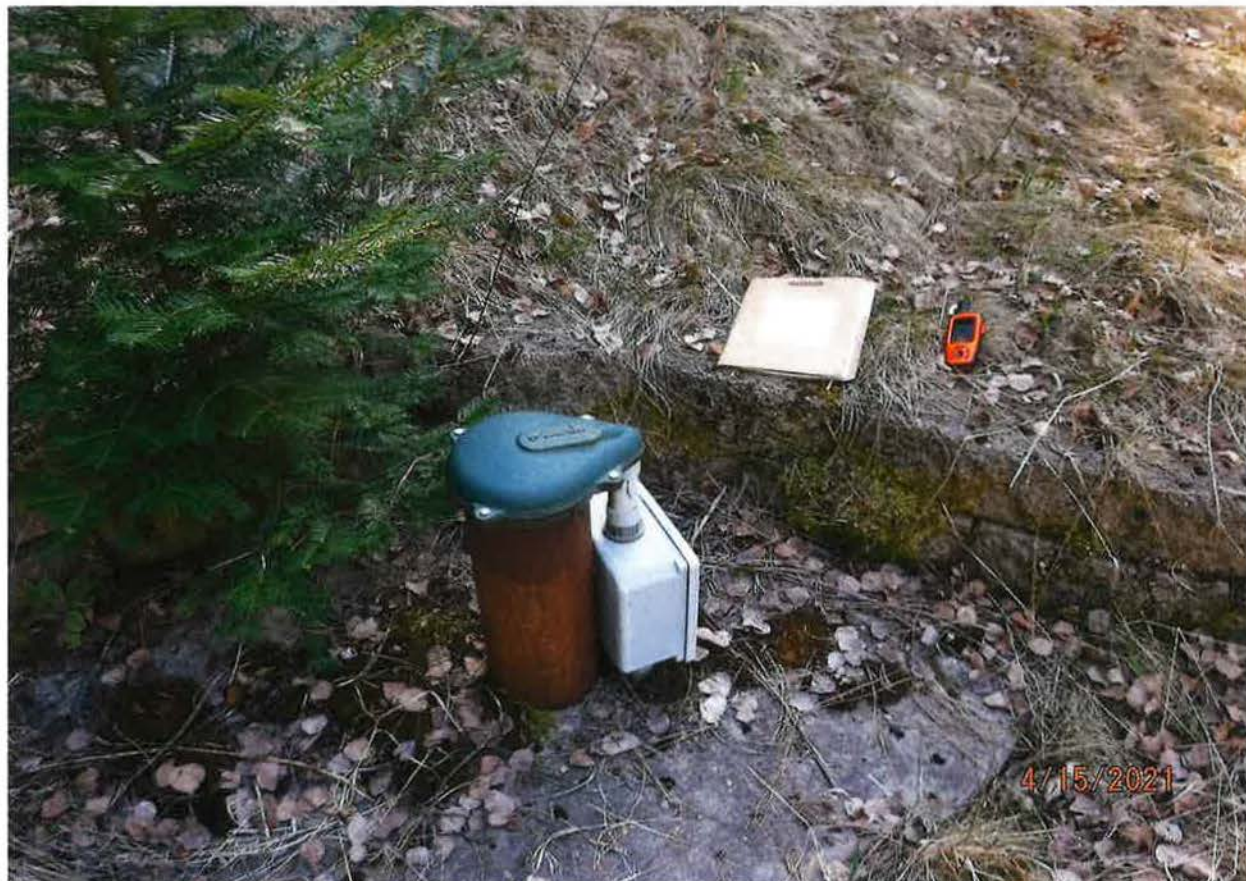
POD - WELL D0028026
