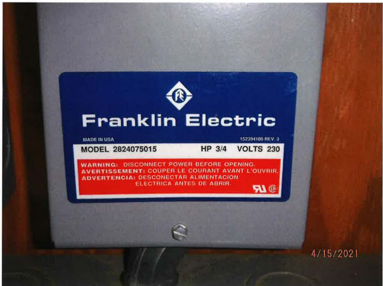
INJECTION WELL D0028065 ¾ HP PUMP INSTALLED
