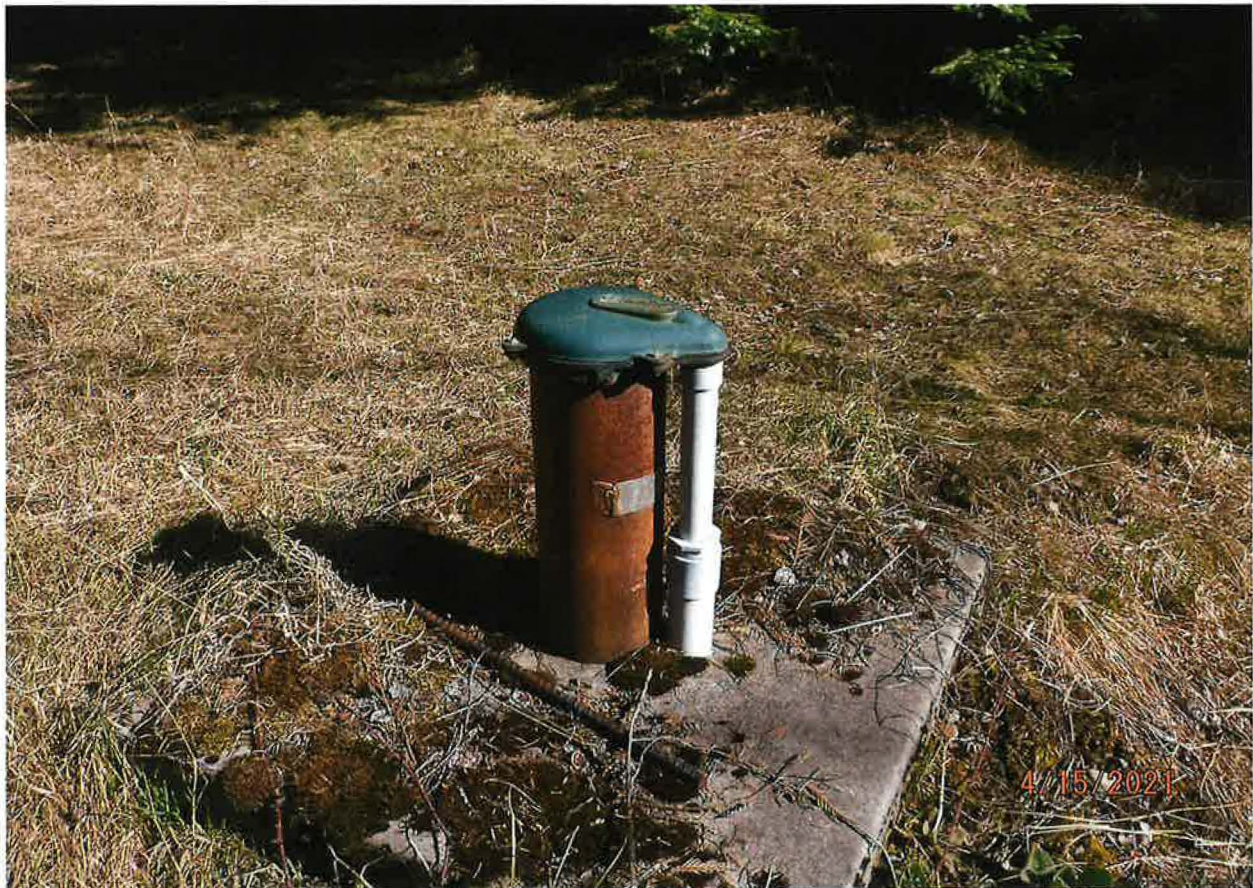
INJECTION WELL -D0028065
