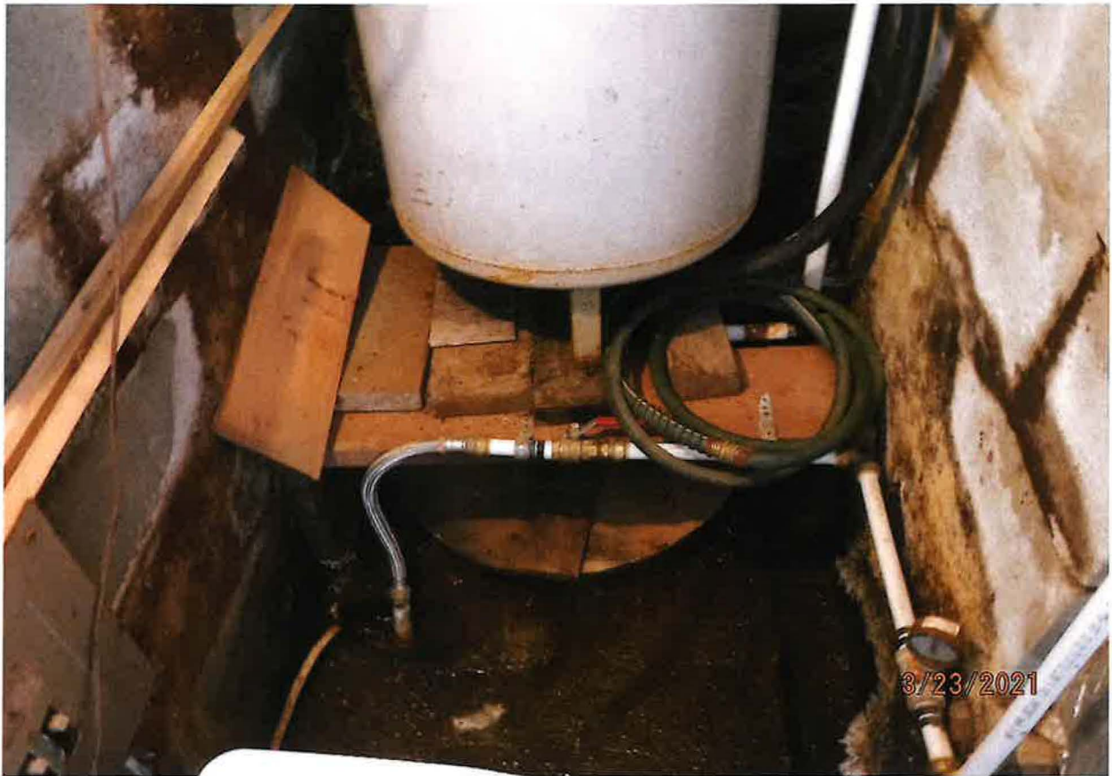
POD – 2 FT CULVERT PLACED 4 FT DEEP IN GROUND TO CAPTURE SPRING WATER
