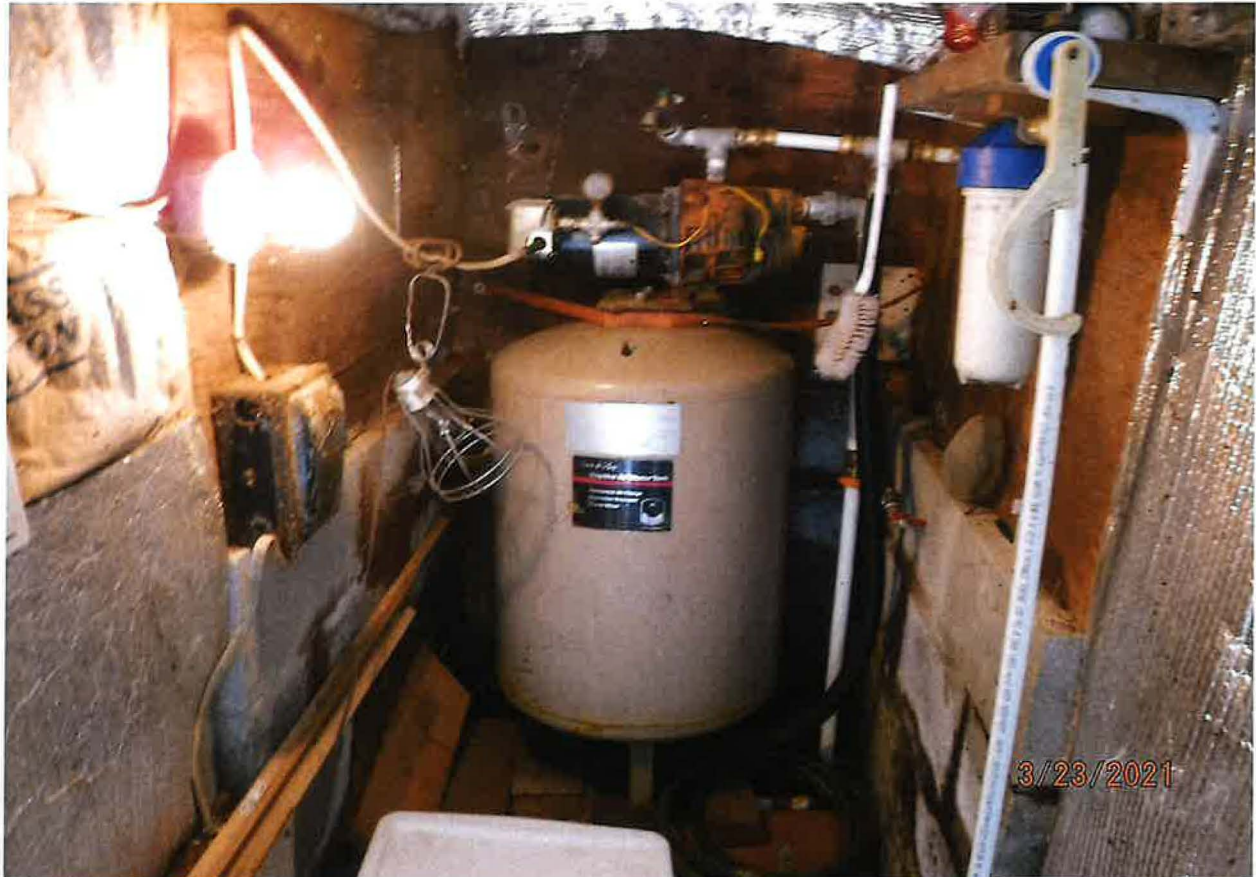
DIVERTING WORKS – 1 INCH POL PIPE FROM PRESSURE TANK TO POU(S)
