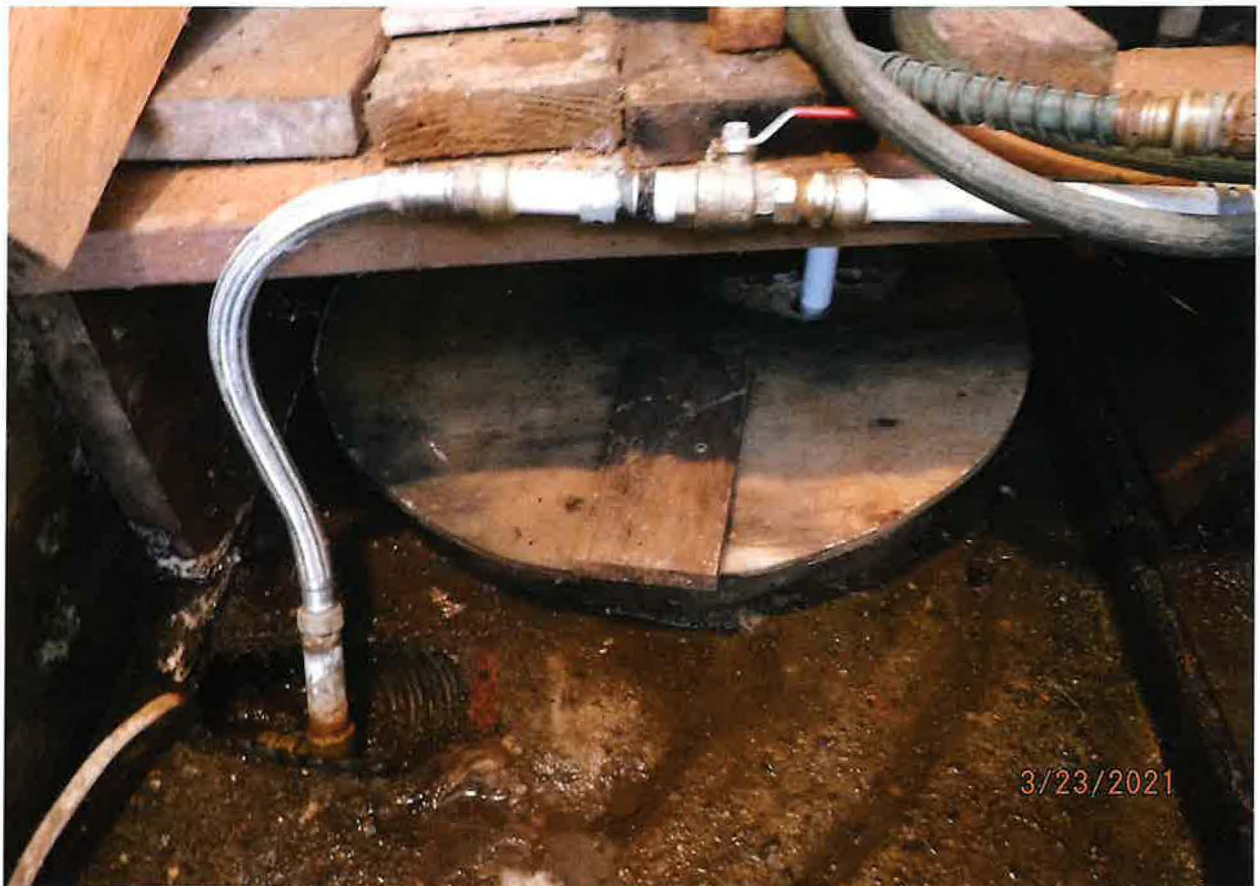
2 FT BY 4 FT CULVERT SERVES AS 24HR IMPOUNDMENT CISTERN
