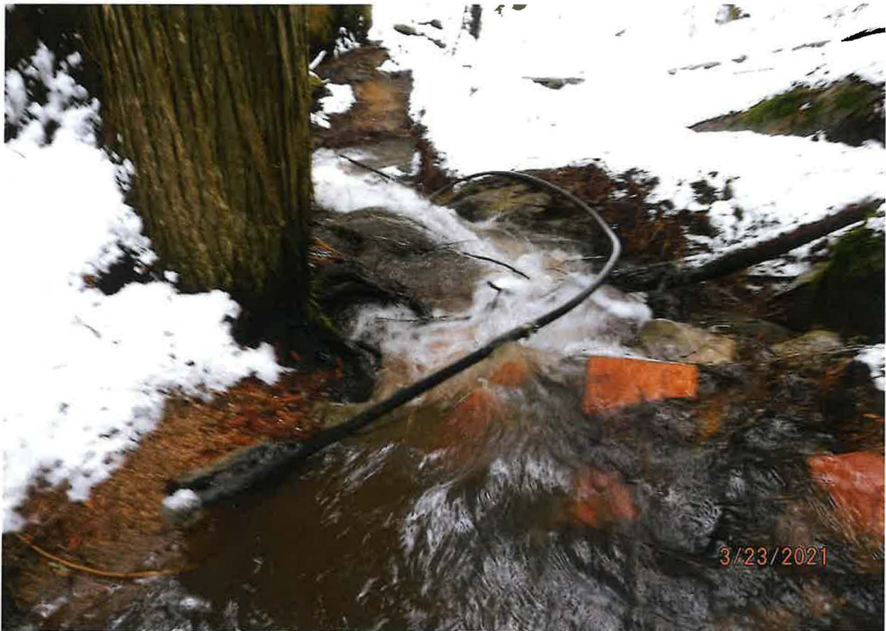
AT POD, 1 INCH PIPE ROUTES DOWN STREAM TO PRESSURE TANK AND FROST FREE HYDRANT
