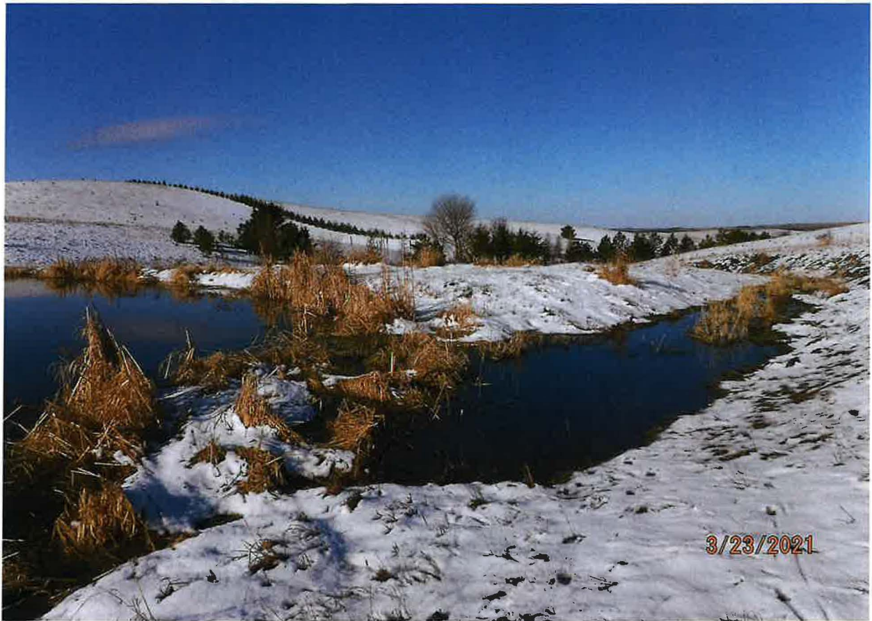
OVERFLOW DISCHARGE CHANNEL AT NORTHWEST CORNER OF POND
