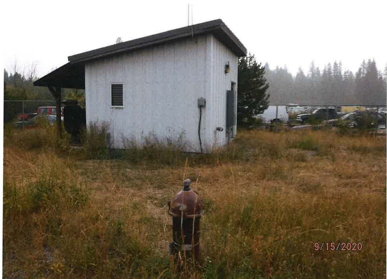
POD – WELL No. 2 95-95-N-0005-000
