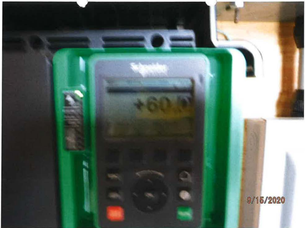
60 PSI SYSTEM OPERATING PRESSURE.
