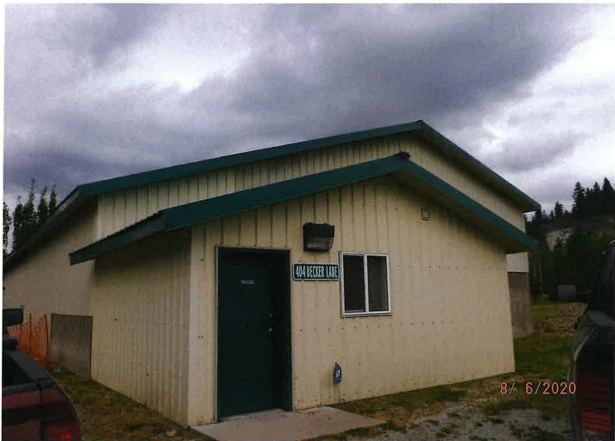
WATER SYSTEM OPERATION BUILDING / SLOW SAND FILTRATION SYSTEM
