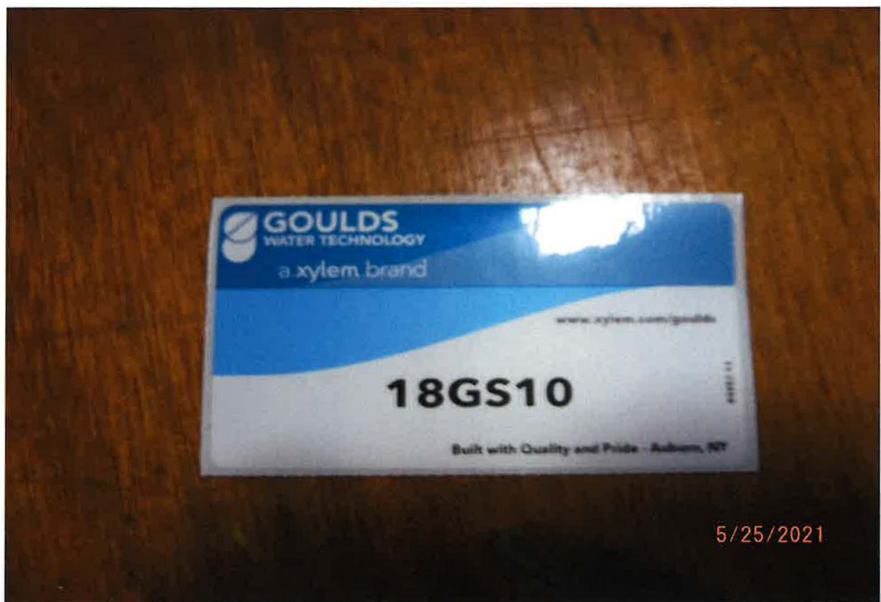
18 GPM, 1 HP GOULDS PUMP INSTALLED IN SYSTEM
