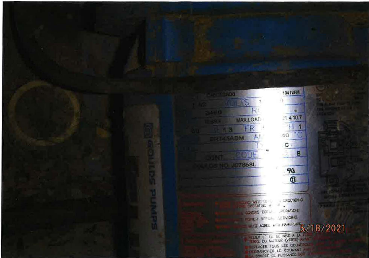
1.5 HP PUMP USED FROM 24 HR IMPOUNDMENT TO PRESSURIZED SPRINKLER SYSTEM
