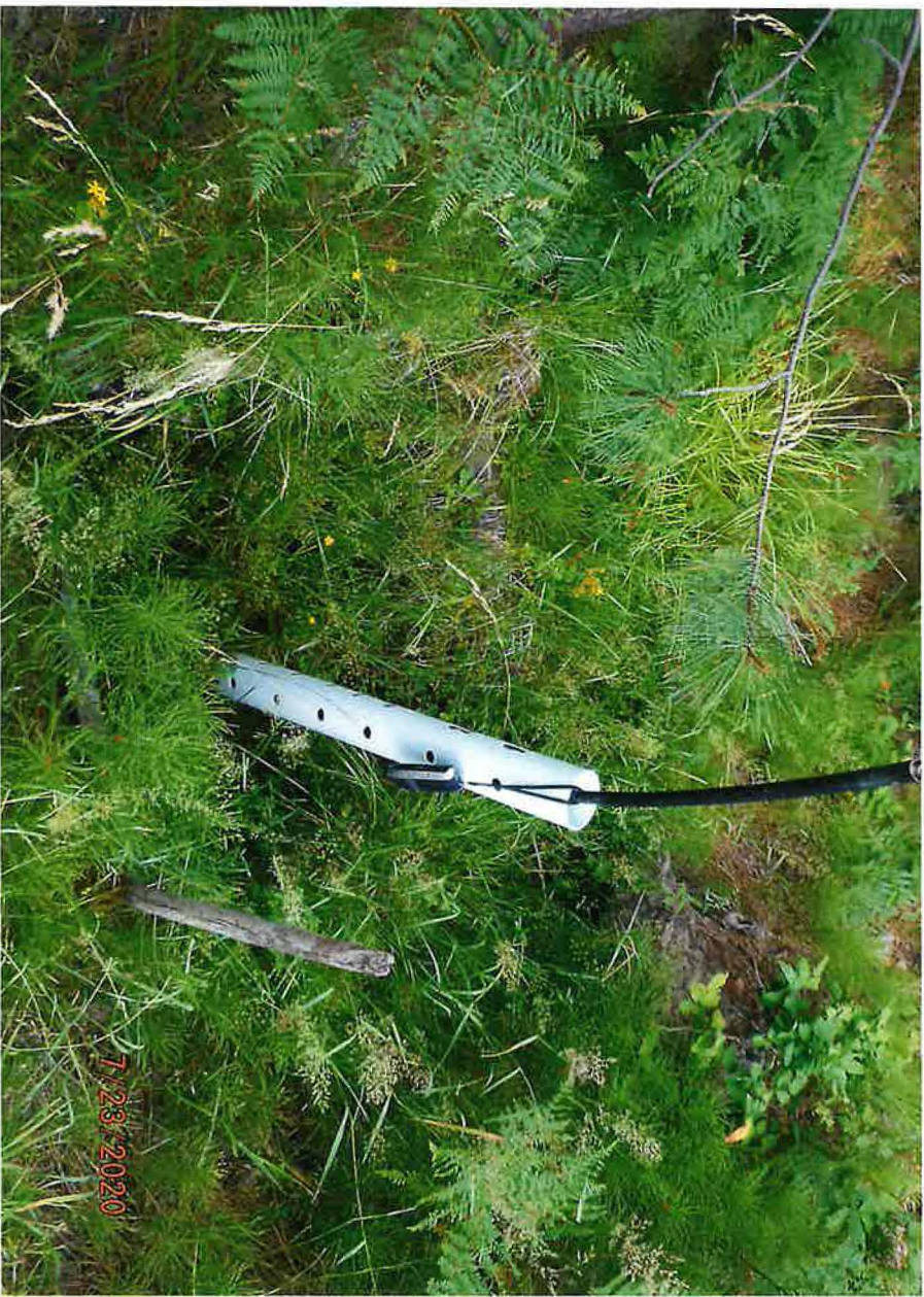
POD – SPRING WITH BURIED SPRING BOX (PIPE ROUTES TO POND No.2)
