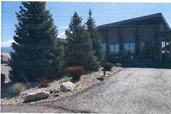
Operations center office building
