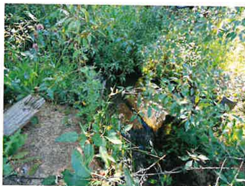
Surface water diversion, old check structure (Lake Irrigation District)
