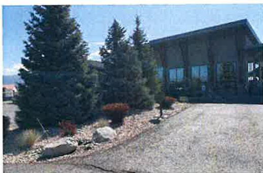
Operations center office building
