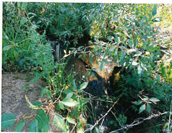
Surface water diversion, old check structure (Lake Irrigation District)
