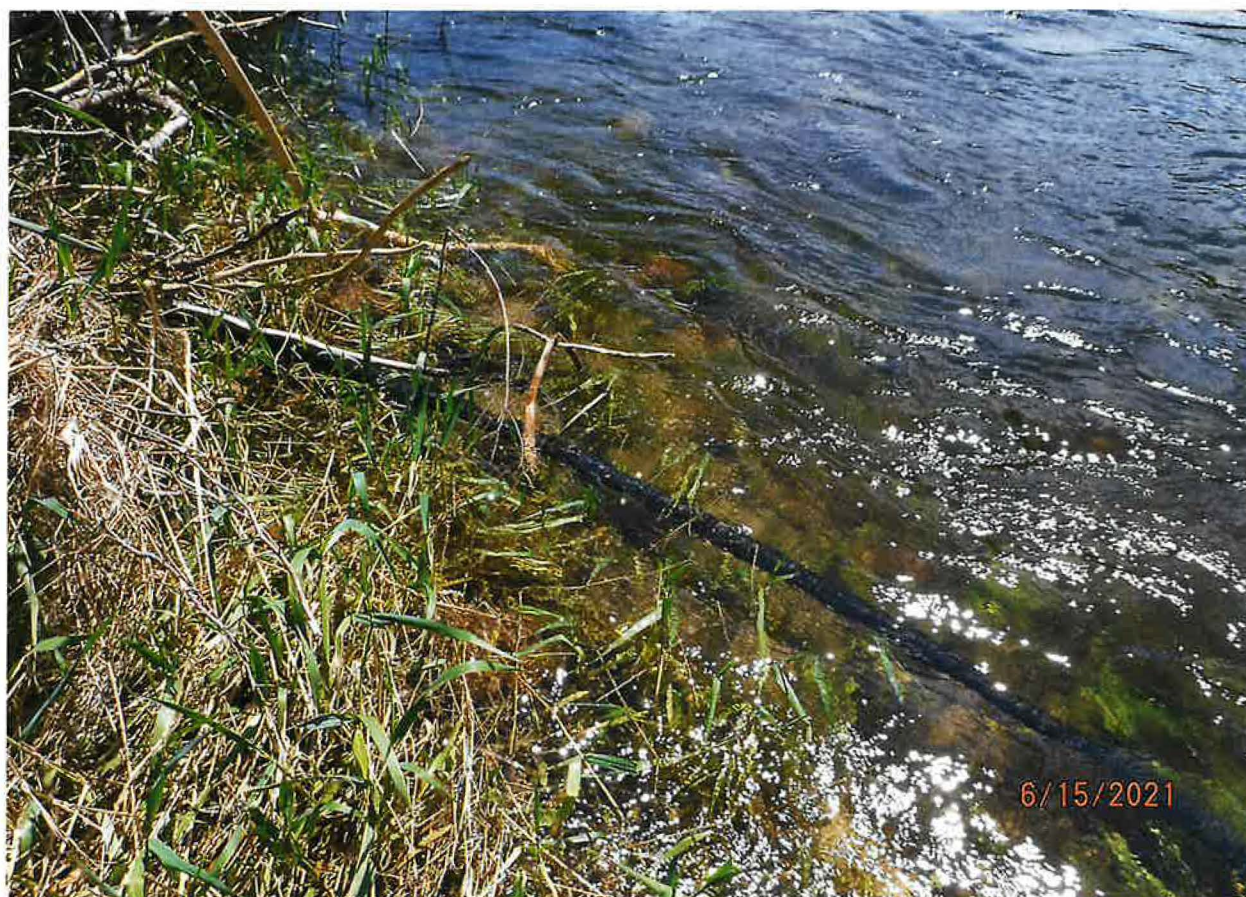
POD – 2 INCH POLY PIPE IN RIVER
