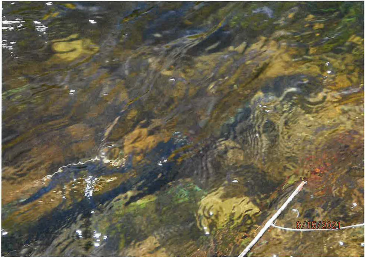
SCREENED INTAKE PIPE IN RIVER
