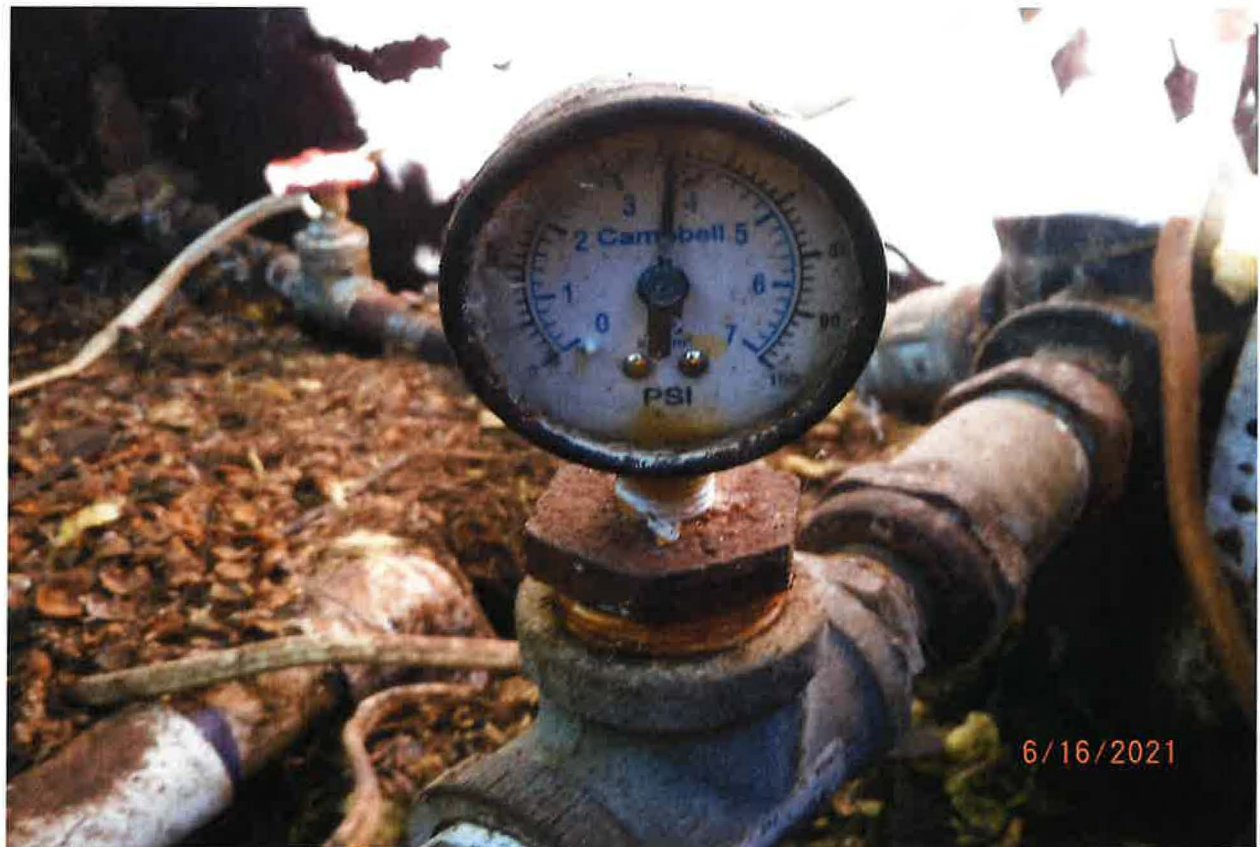
50 PSI SYSTEM OPERATING PRESSURE
