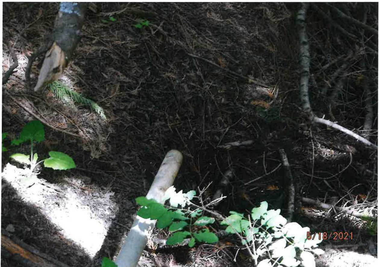
OVERFLOW PIPE FROM RESERVOIR (NOT FLOWING DURING FIELD EXAM)
