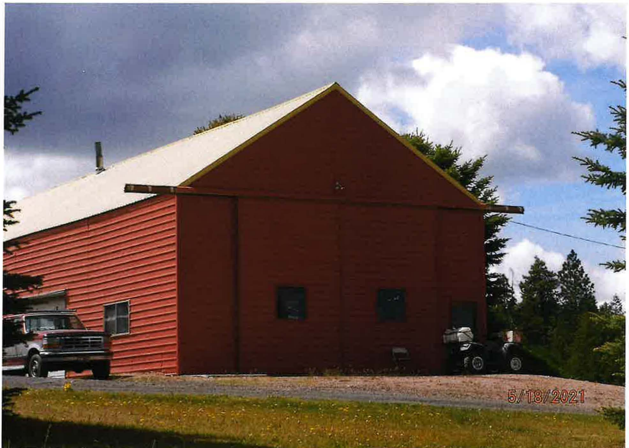
DOMESTIC POU – SHOP HAS WATER LINE AND RESTROOM FACILITIES
