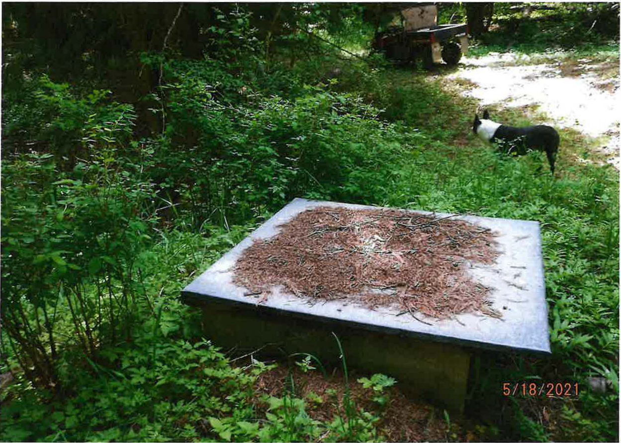
WATER FROM POD PIPED DOWNHILL 20 YARDS TO CONCRETE RESERVOIR
