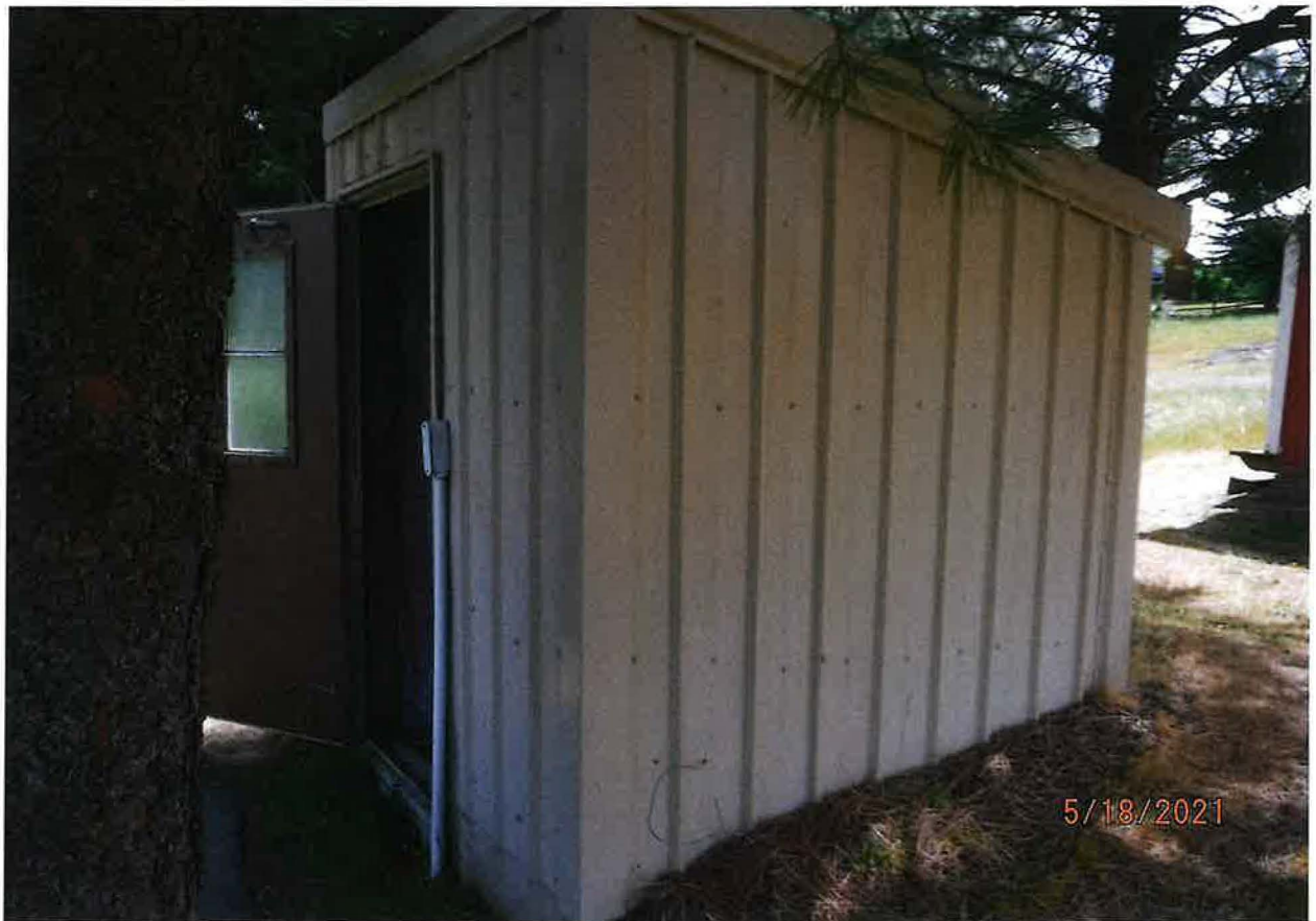
SMALL PUMP HOUSE LOCATED NW OF MAIN HOUSE
