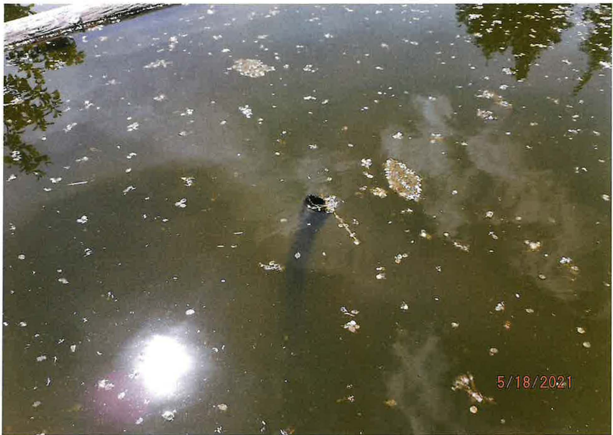
OVERFLOW PIPE FROM STOCKWATER RESERVOIR
