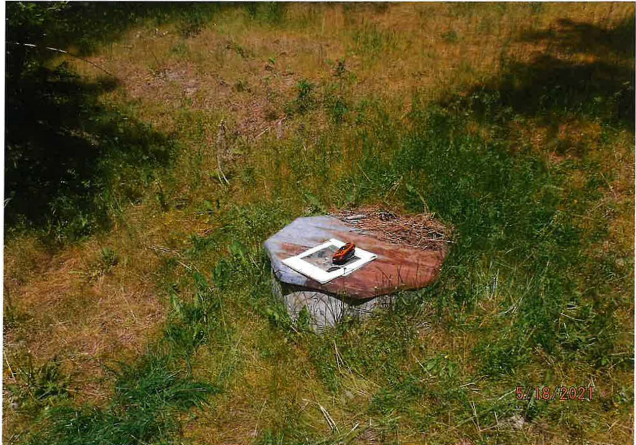
POD – VERTICAL CULVERT CAPTURES SPRING WATER BEFORE PIPING DOWNHILL TO POU
