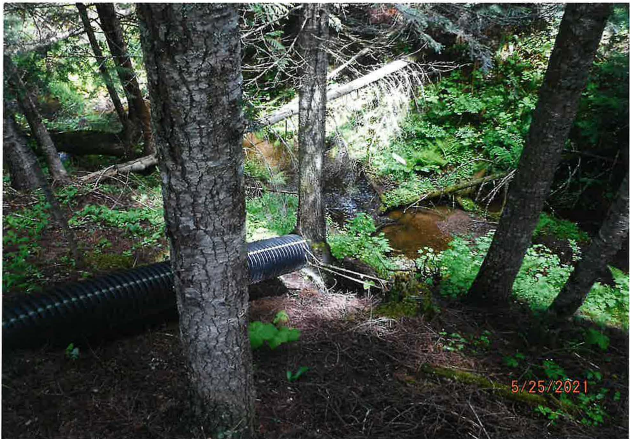
OVERFLOW WATER FROM POND FLOWS INTO MIRROR CREEK
