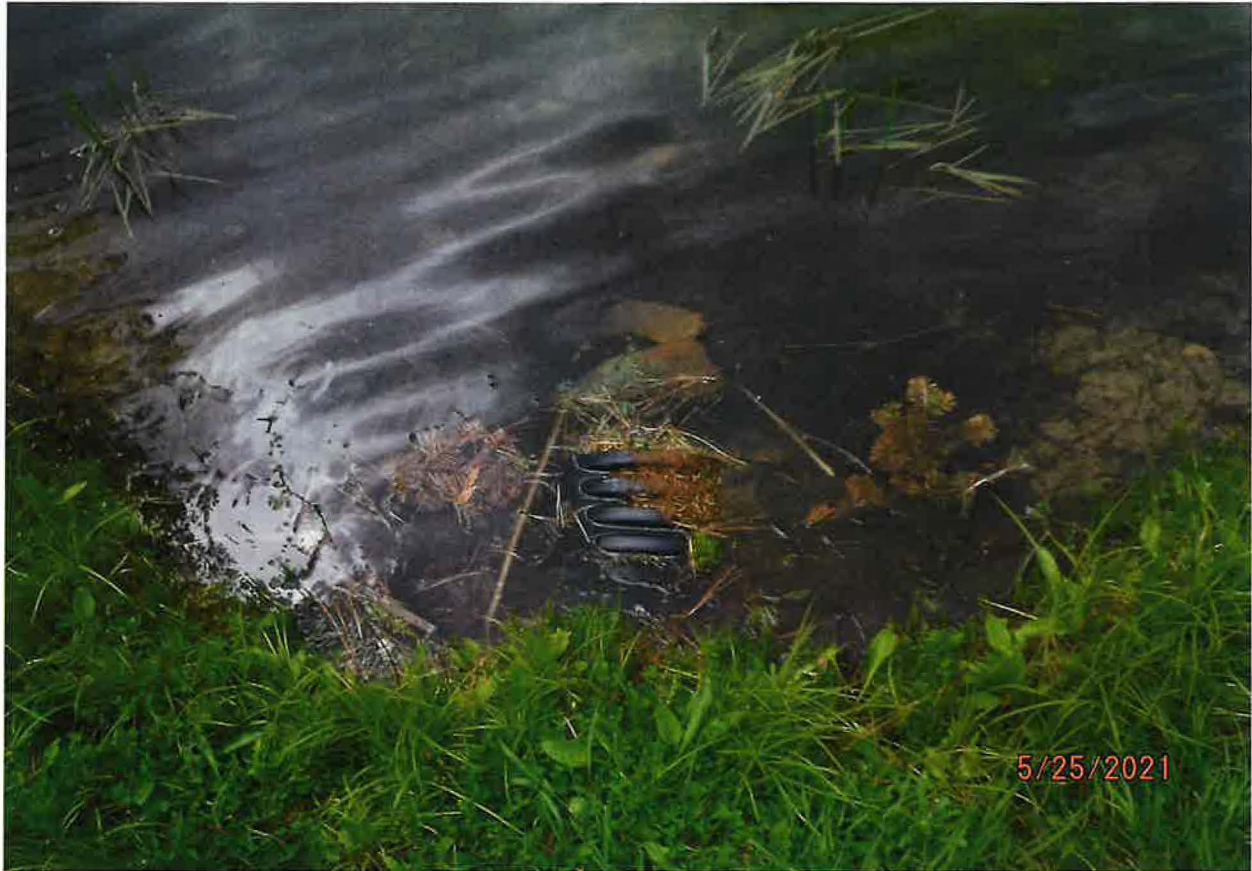
SCREENED OVERFLOW DISCHARGE CORRUGATED PIPE
