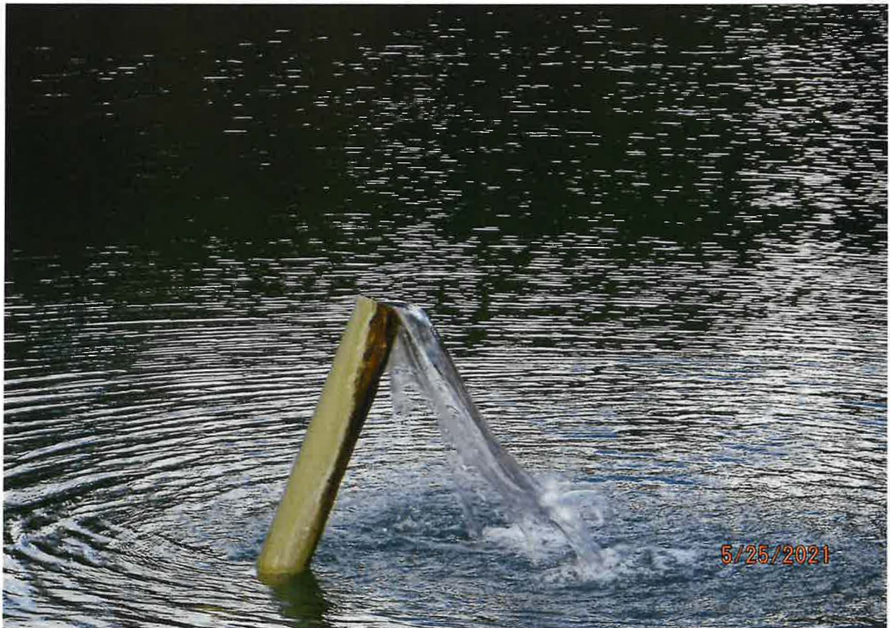
INFLOW FROM SPRING SOURCE – 1400 FT RUN OF 4" PVC PIPE TO VERTICAL RISER IN POND
