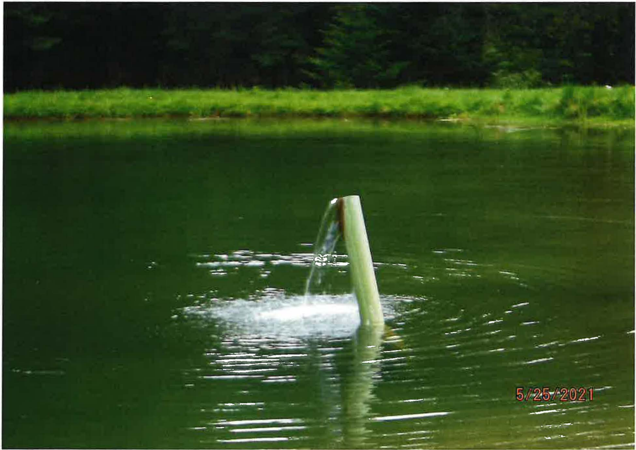
INFLOW FROM SPRING SOURCE – 1400 FT RUN OF 4" PVC PIPE TO VERTICAL RISER IN POND
