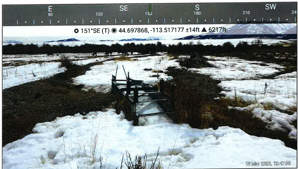
Figure 5: Photo of the lower ditch, measuring flume in ditch, facing upstream towards the point of diversion.
