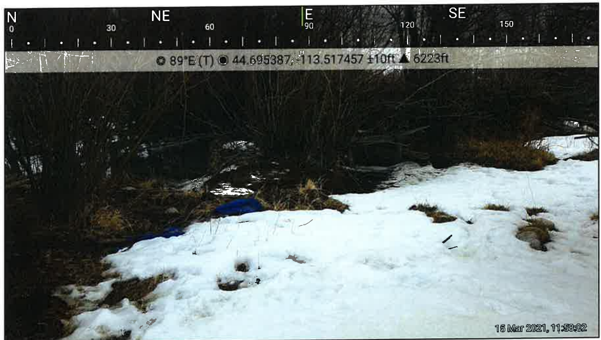
Figure 4: Photo of lower point of diversion check structure and diversion works.
