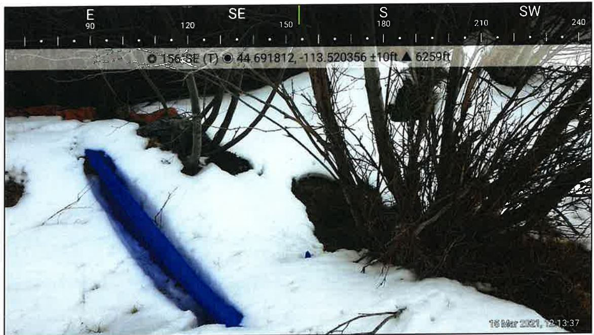
Figure 2: Photo of check dam at upper point of diversion.
