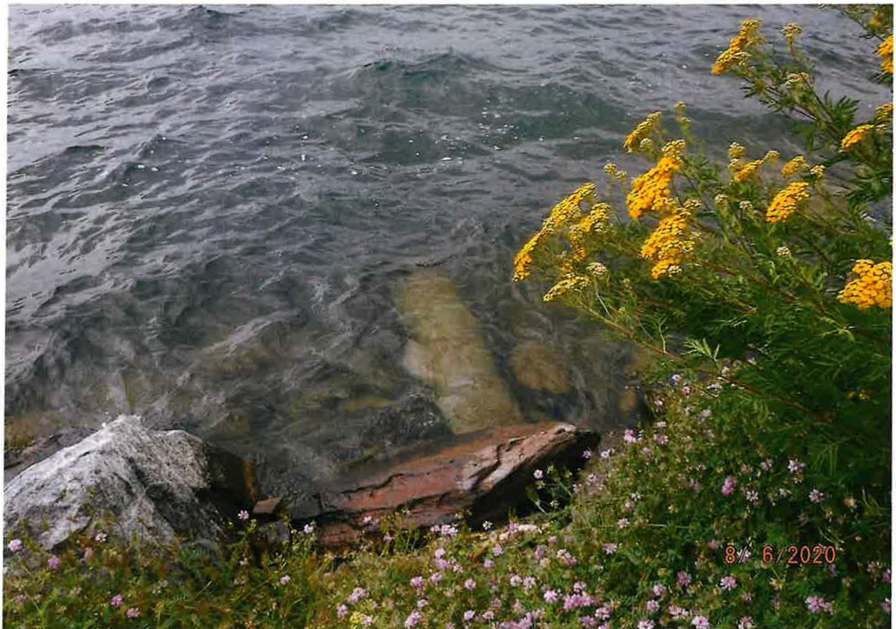
AESTHETIC FLOW THROUGH PIPE – DISCHARGES BACK TO PEND OREILLE RIVER
