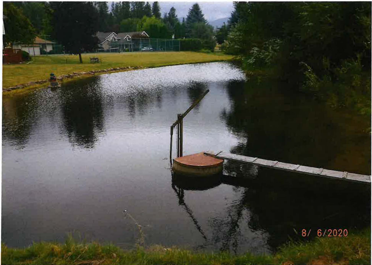
AESTHETIC & AESTHETIC STORAGE POU – DISCHARGE PIPE CONTROL SYSTEM BACK TO RIVER
