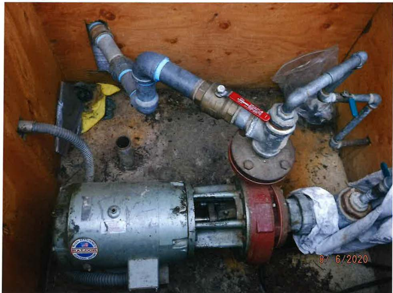
POD - 15 HP PUMP WITH PIPE IN RIVER
