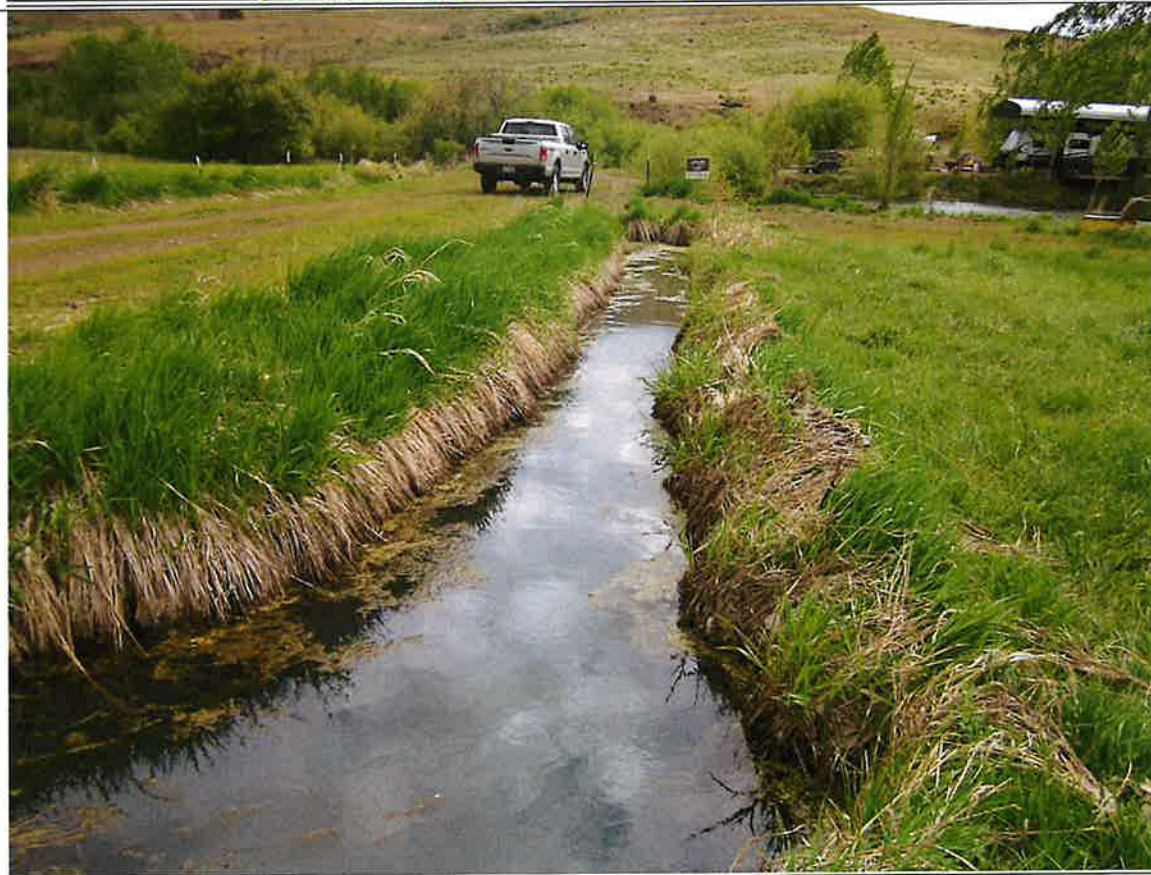
Figure 4. A ditch parallels the south side of the access road to collect spring water. At the time of the field exam spring flow matched the pond level.
