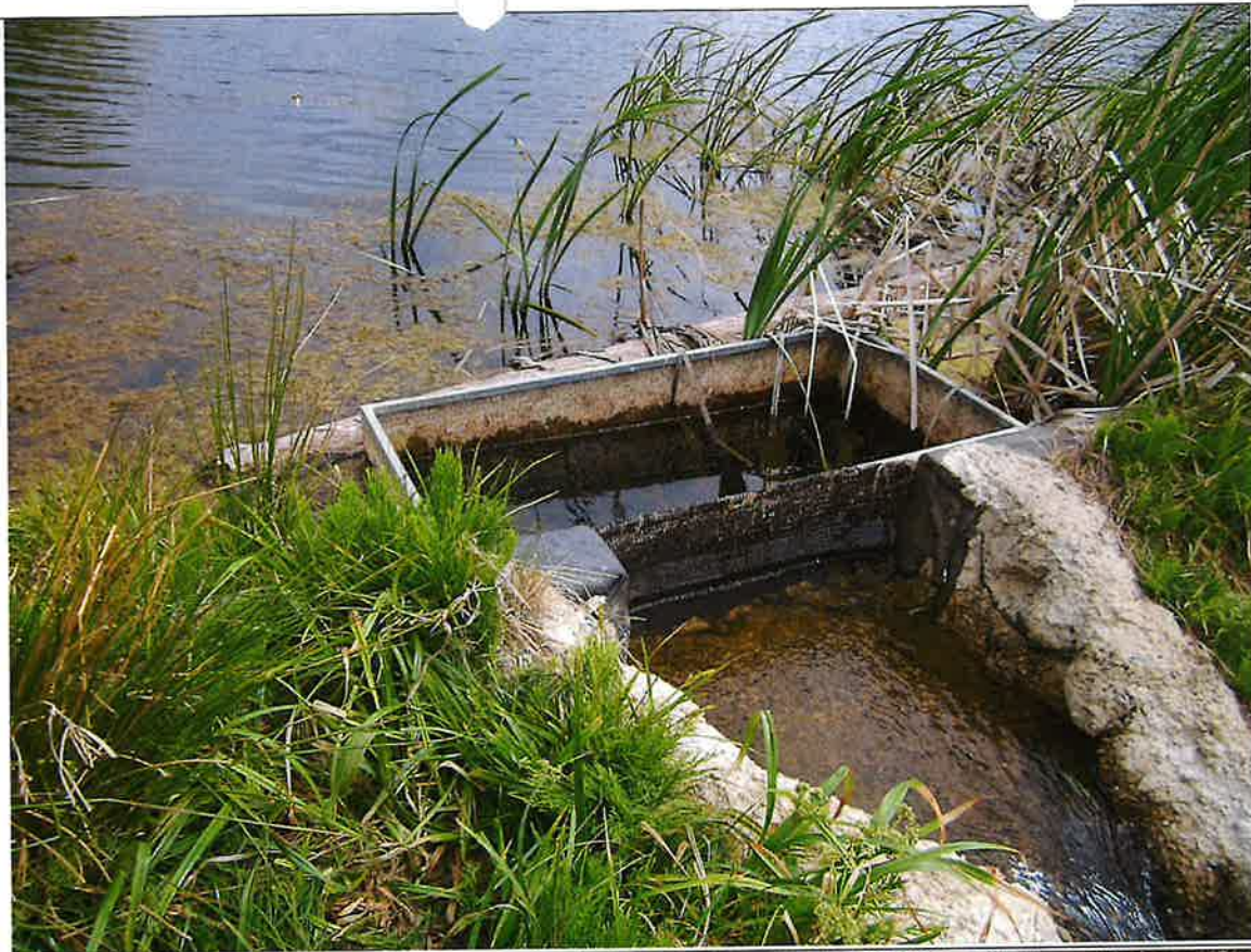
Figure 5. Screened outflow at the south end of the pond.
