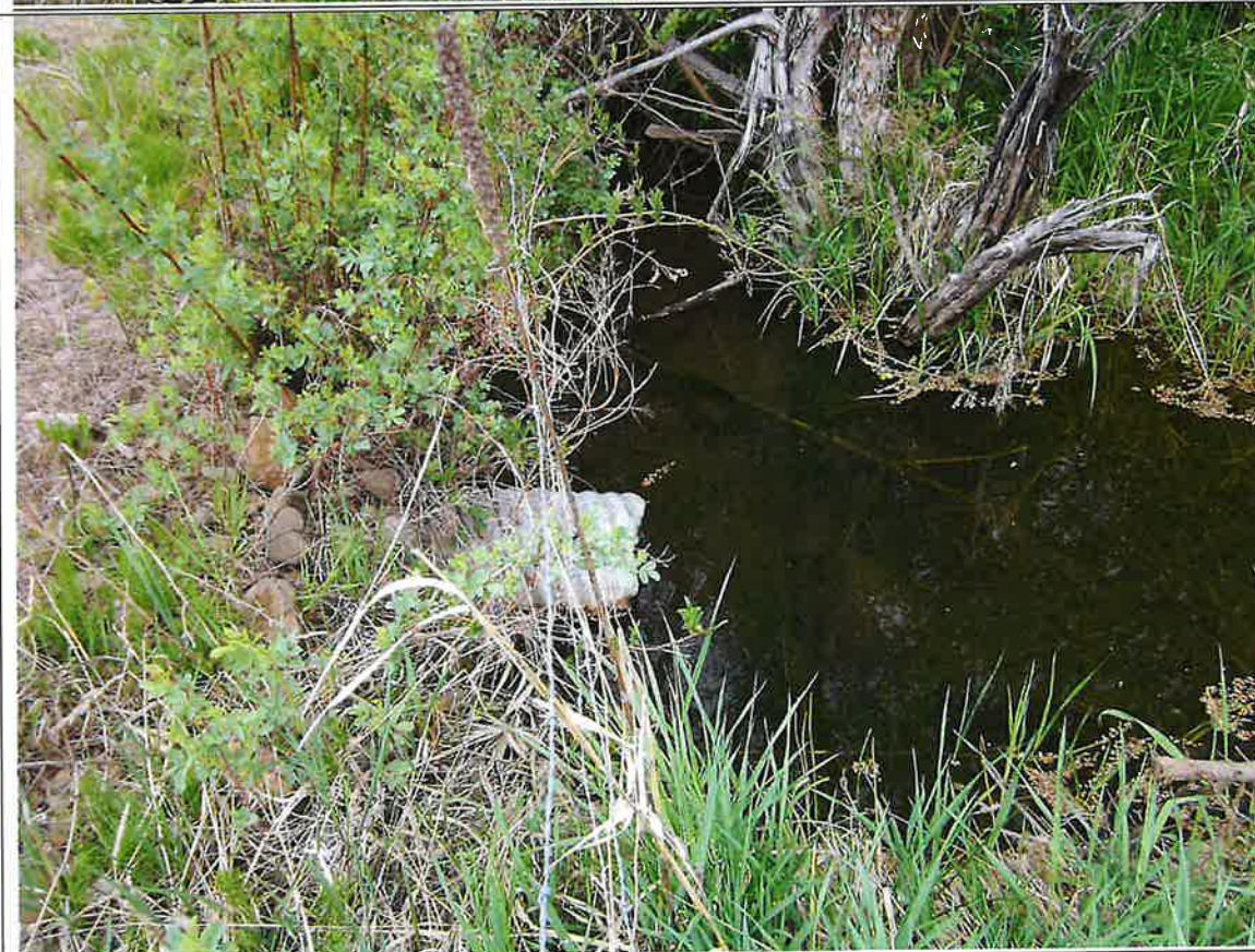
Figure 2. Collected waster enters the Appleby property through an 8 inch culvert under the access road.
