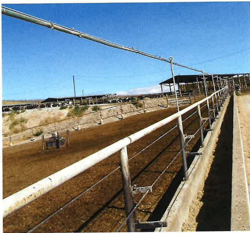
Figure 15 Mistlers Attached to Railing & Used Seasonally
