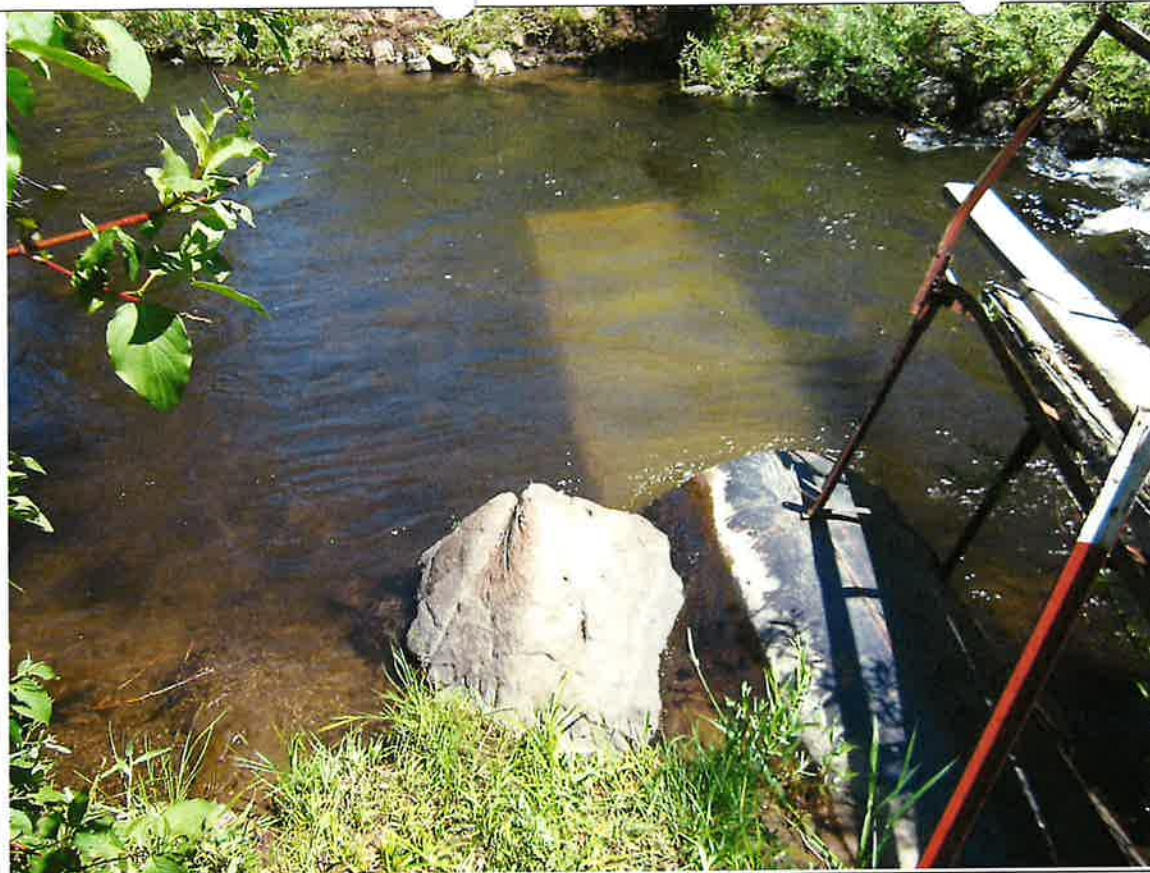
Figure 1. Point of diversion from Second Fork Squaw Creek into 18" culvert
