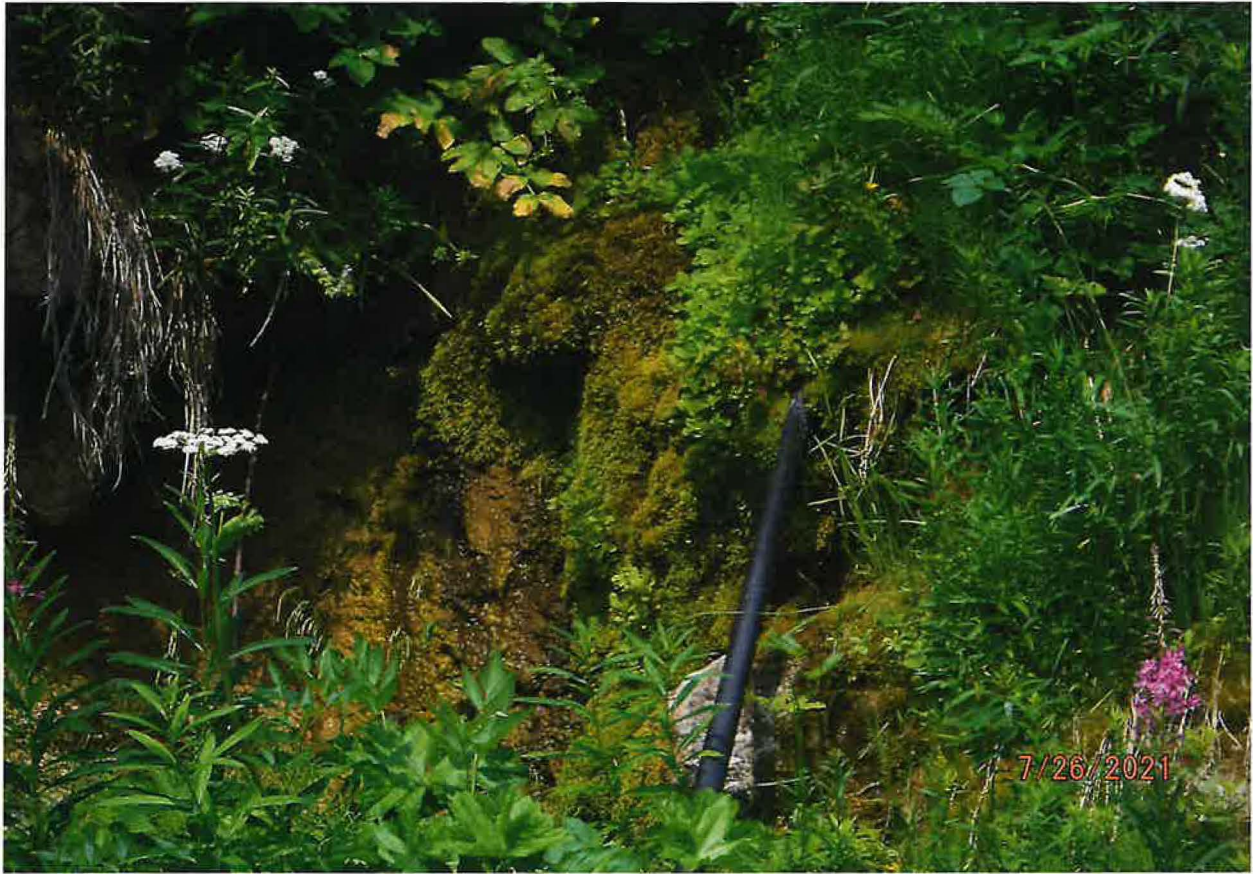
POD – 1.5 INCH POLY PIPE ROUTED DOWN EMBANKMENT TO MINE AREA
