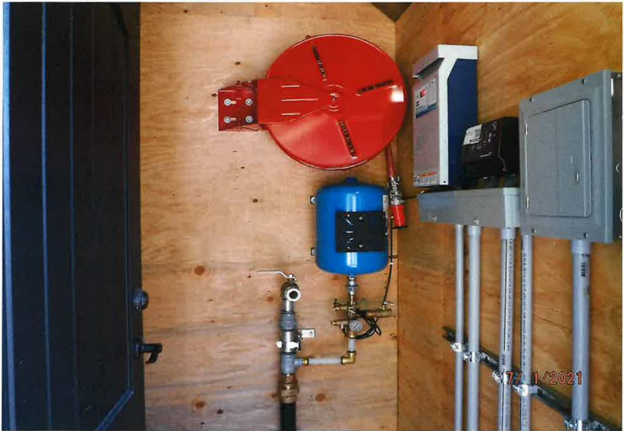
FIRE PROTECTION -- 2 OF 2 FIRE HOSE HOOK UPS WITH REEL
