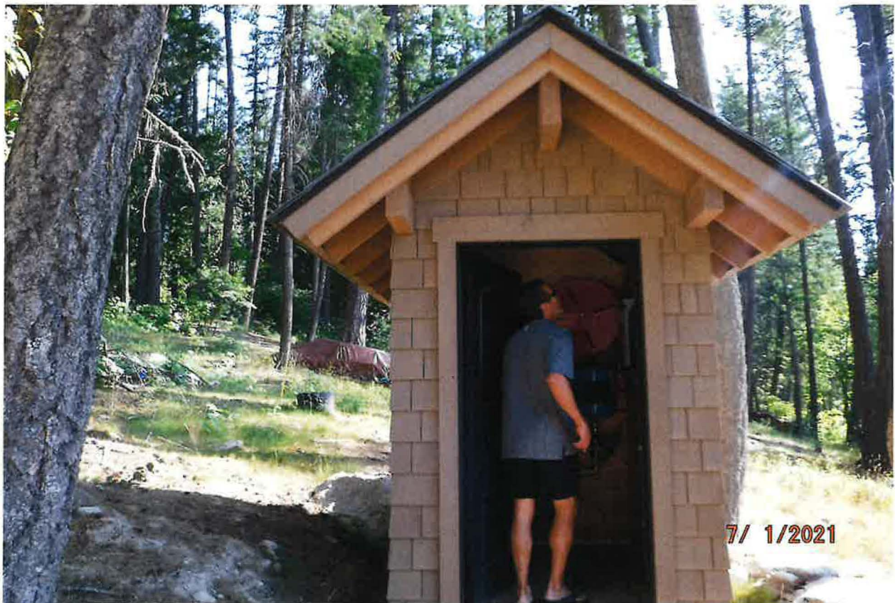
SMALL PUMP HOUSE LOCATED UPGRADE FROM HOME
