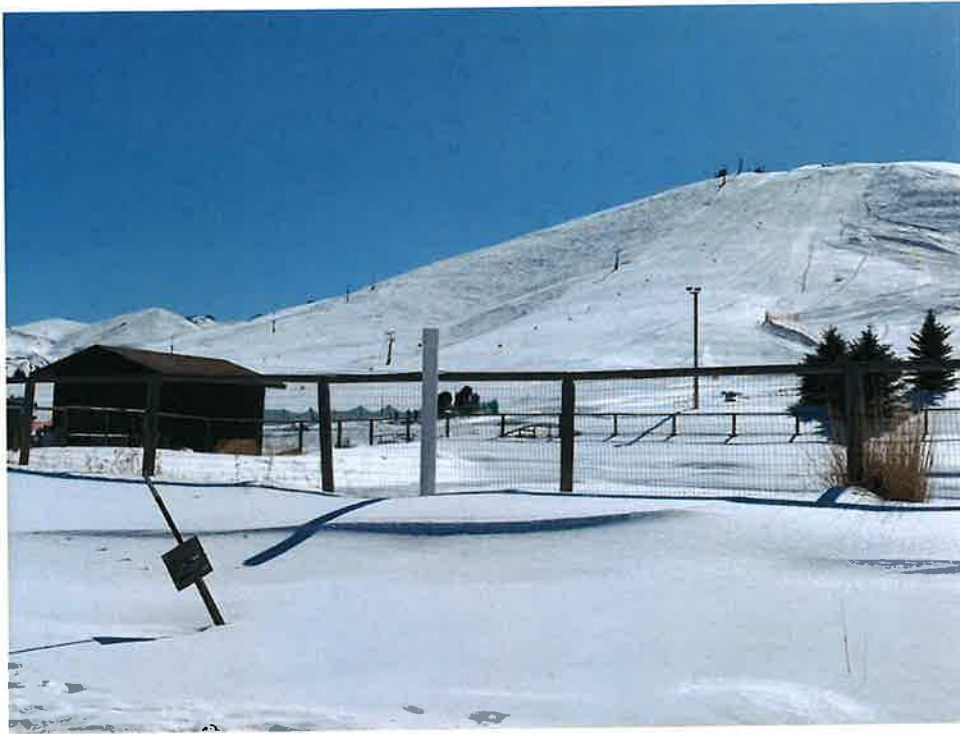
Photo 11: Looking south at ski facility, storage pond, pump house, and vertical wet hydrant connection.
