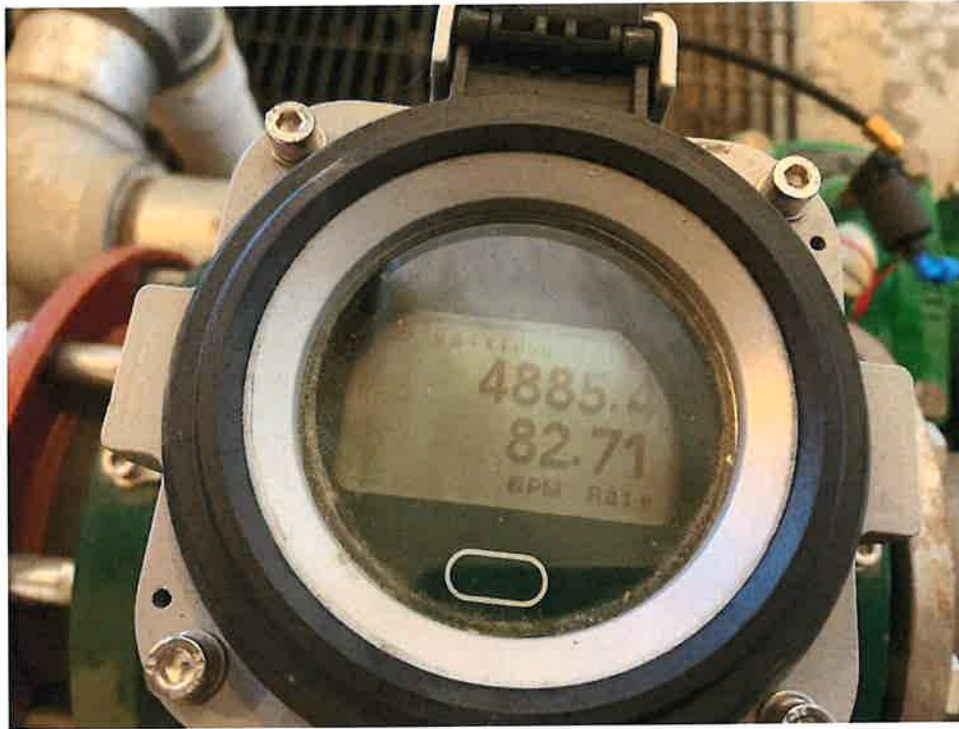
Photo 5: Magnetic flow meter on well inlet line in pump house during 13-minute flow test.
