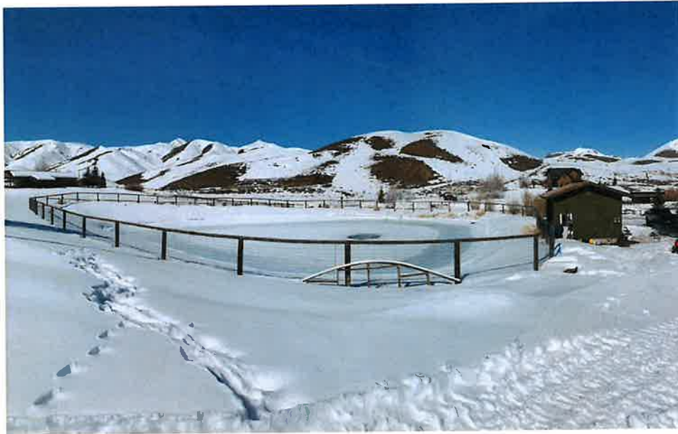
Photo 7: Storage pond and pump house looking north on March 4 th 2021.
