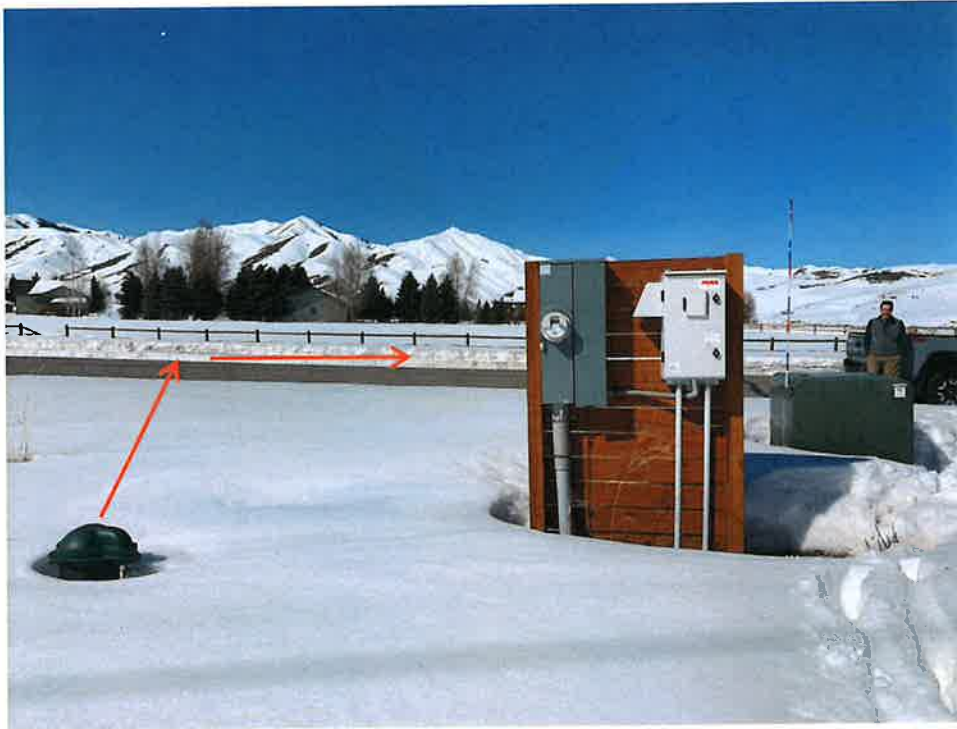
Photo 1: Well head, drive and power, looking west. Arrows denote path of buried 4" delivery line.
