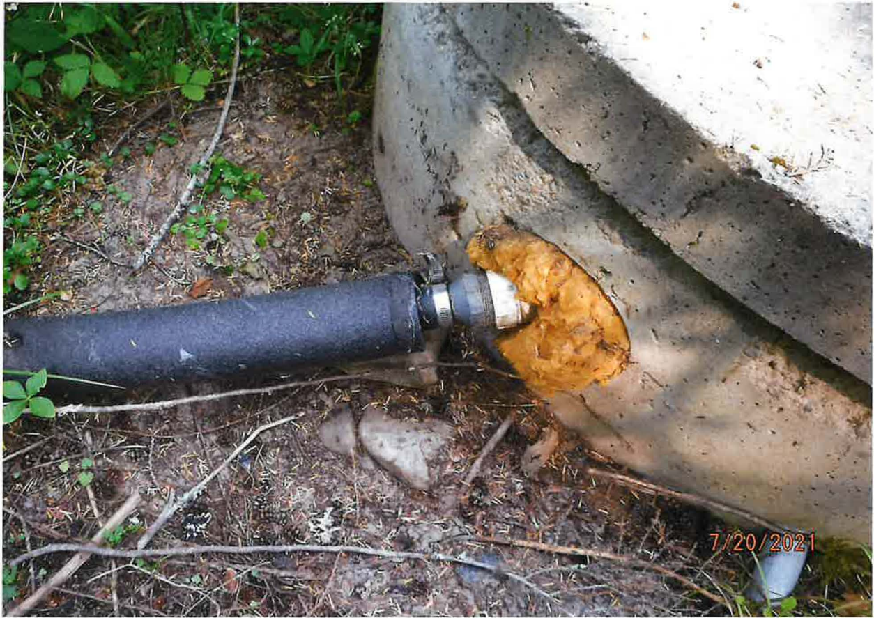
1.5 INCH SERVICE LINE ROUTED FROM POD-TO-POU
