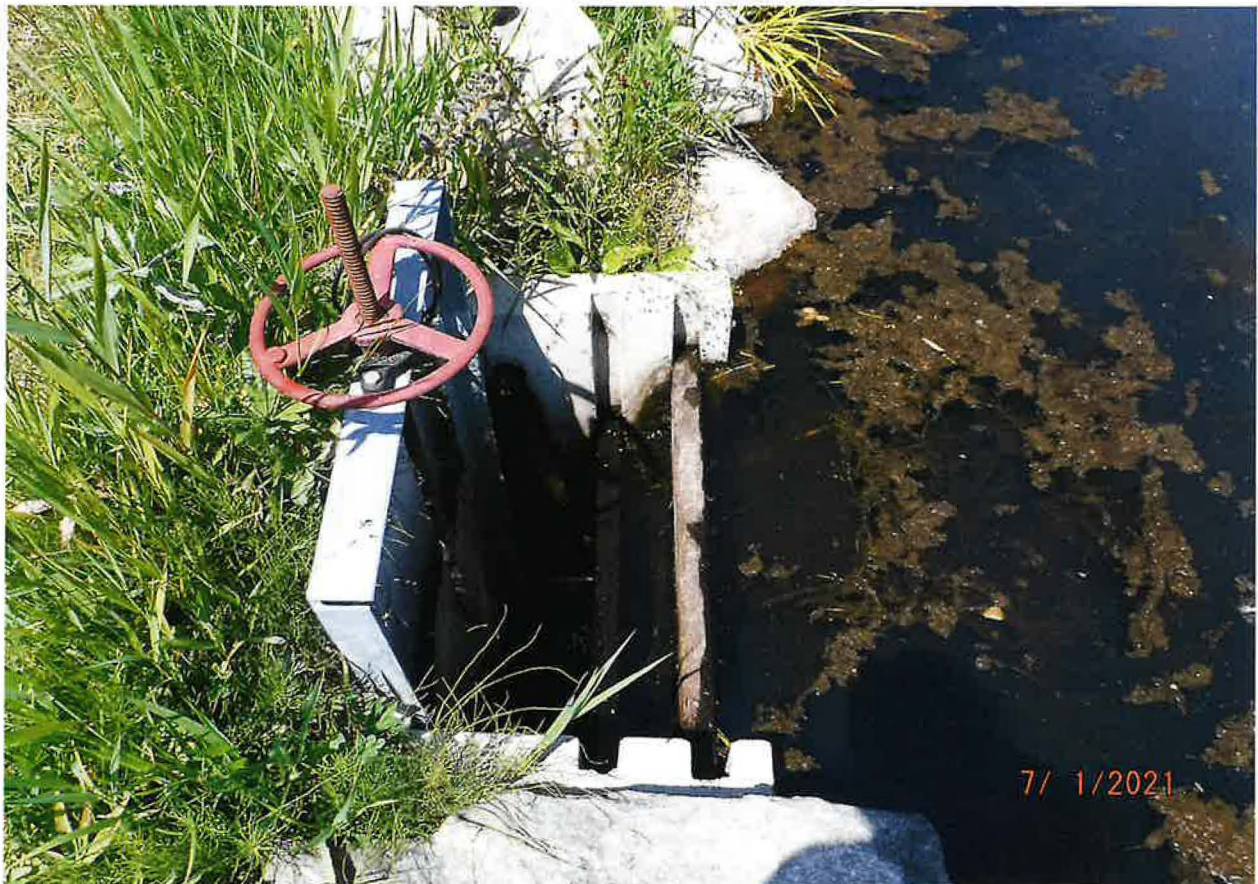
POD – EARTHEN POND DAM WITH WEIR HEADGATE DEVICE INSTALLED
