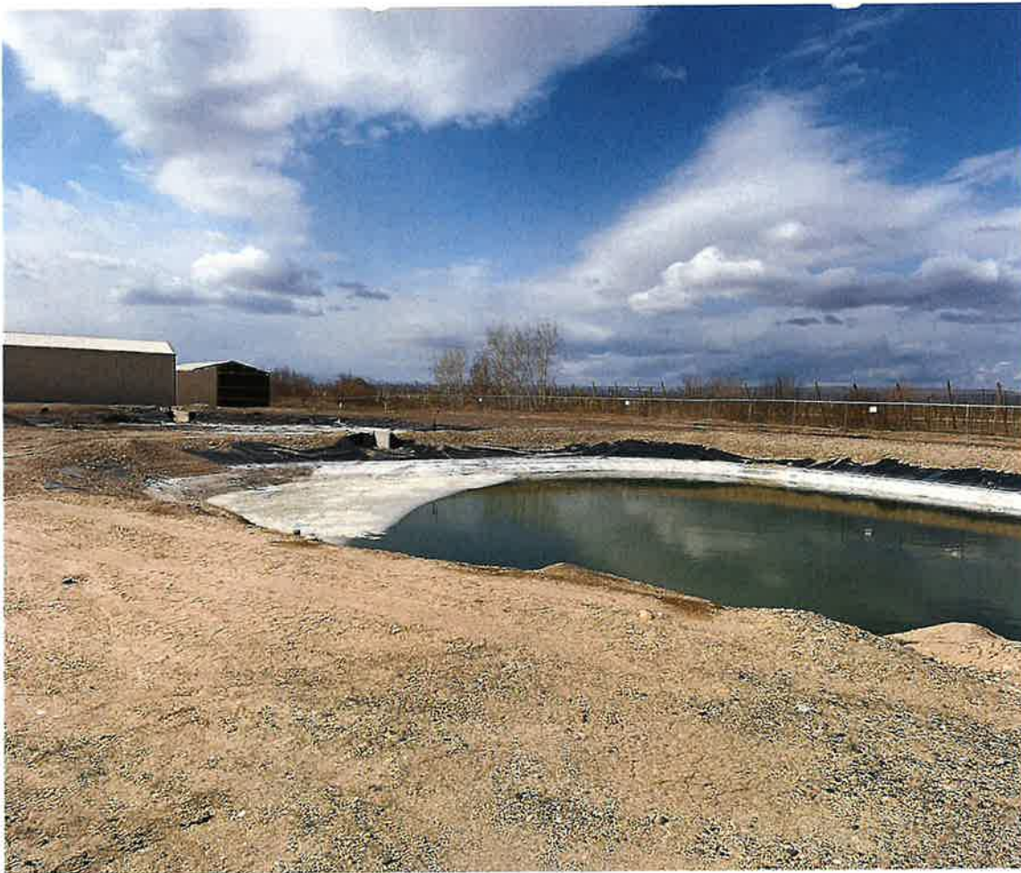
Fig. 21 – View of the two western settling ponds. Settling ponds are reserved for use when DAF building is not operating.
