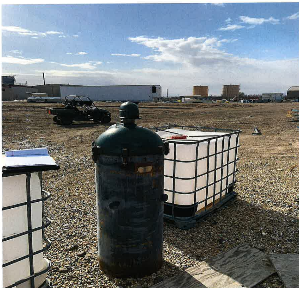
Fig. 2 – Well tag ID #D0064298 has a 14" casing from 2-385 ft, 12" casing from 376- 385 ft, and 8" casing from 385- 401; 431-432 ft bsl.
