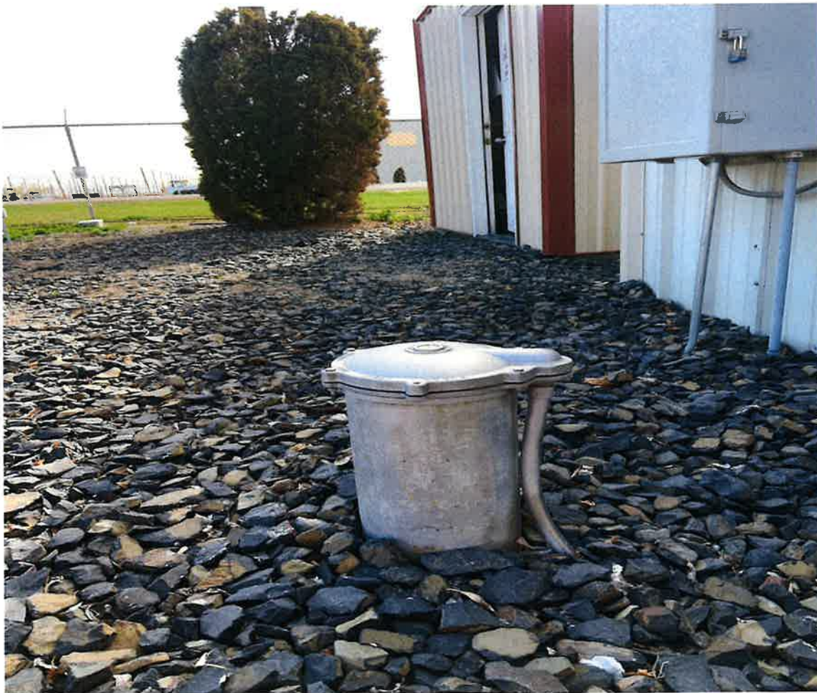
Fig. 8 – Well with no metal tag to the east of the plant. The well log submitted with the application states this is an 8" cased well drilled in 1987.
