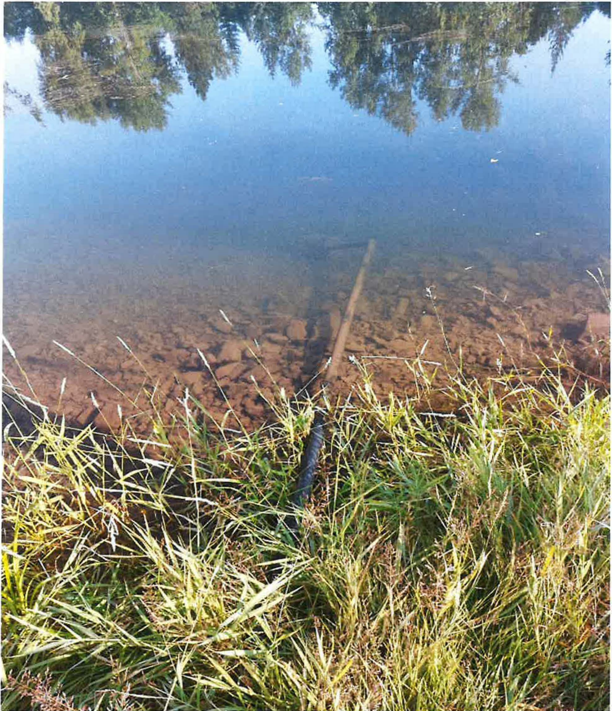
POD – 20FT OF 2" SCREENED (FILTER ENCASED) INTAKE PIPE IN RIVER
