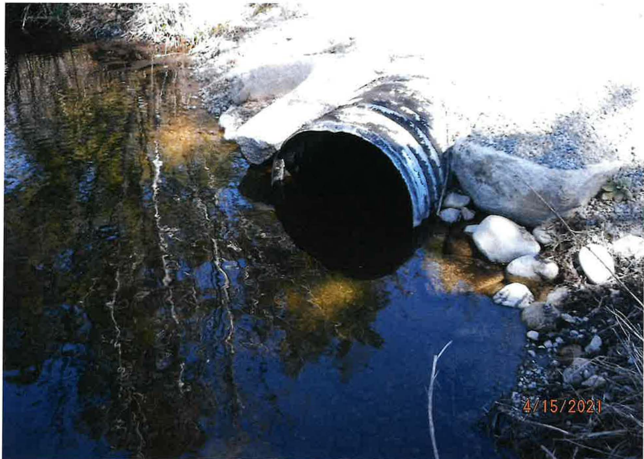
POD – POND SIDE OF CREEK DIVERSION PIPE (4/15/2021)
