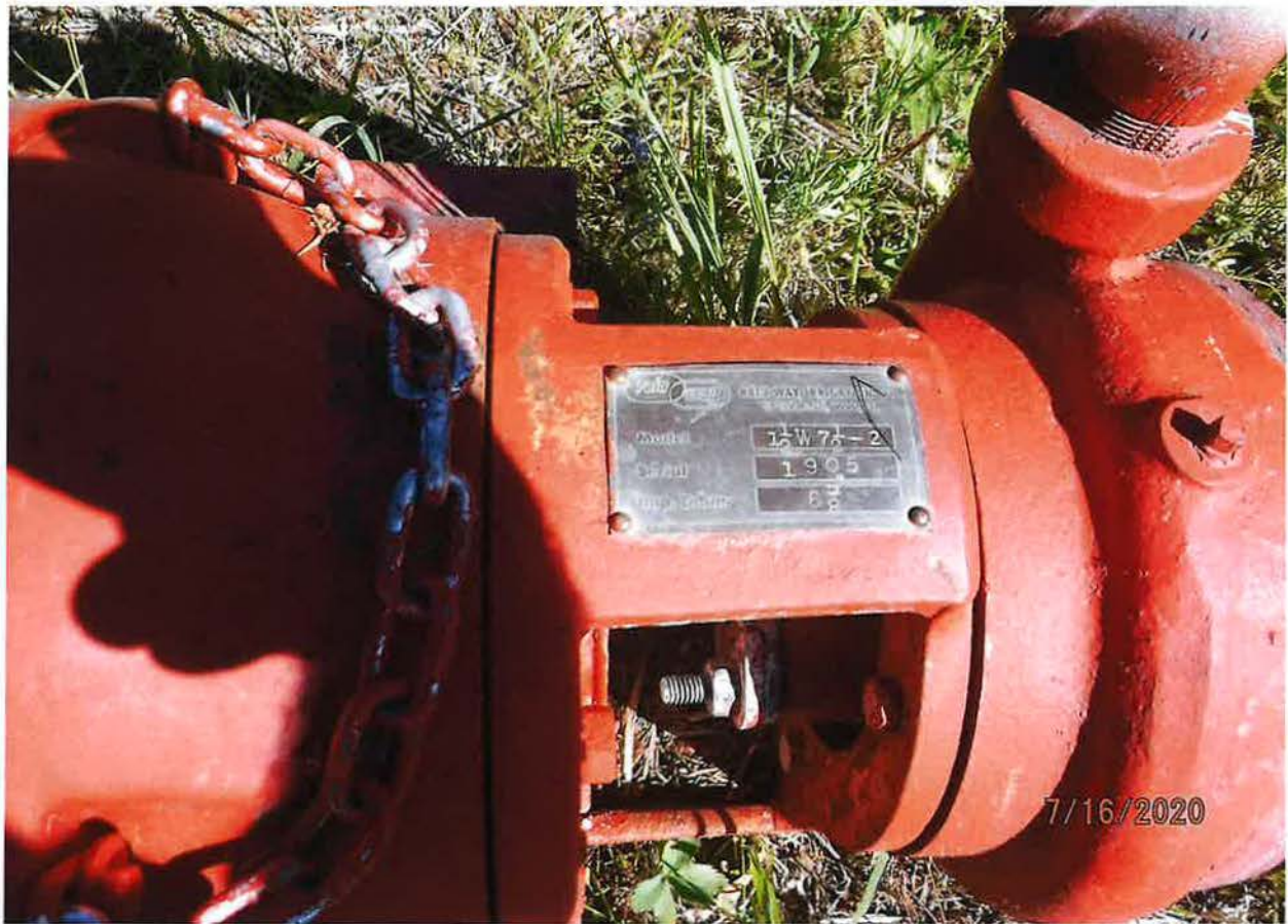
7.5 HP PUMP USED ON IRRIGATION FROM STORAGE SYSTEM
