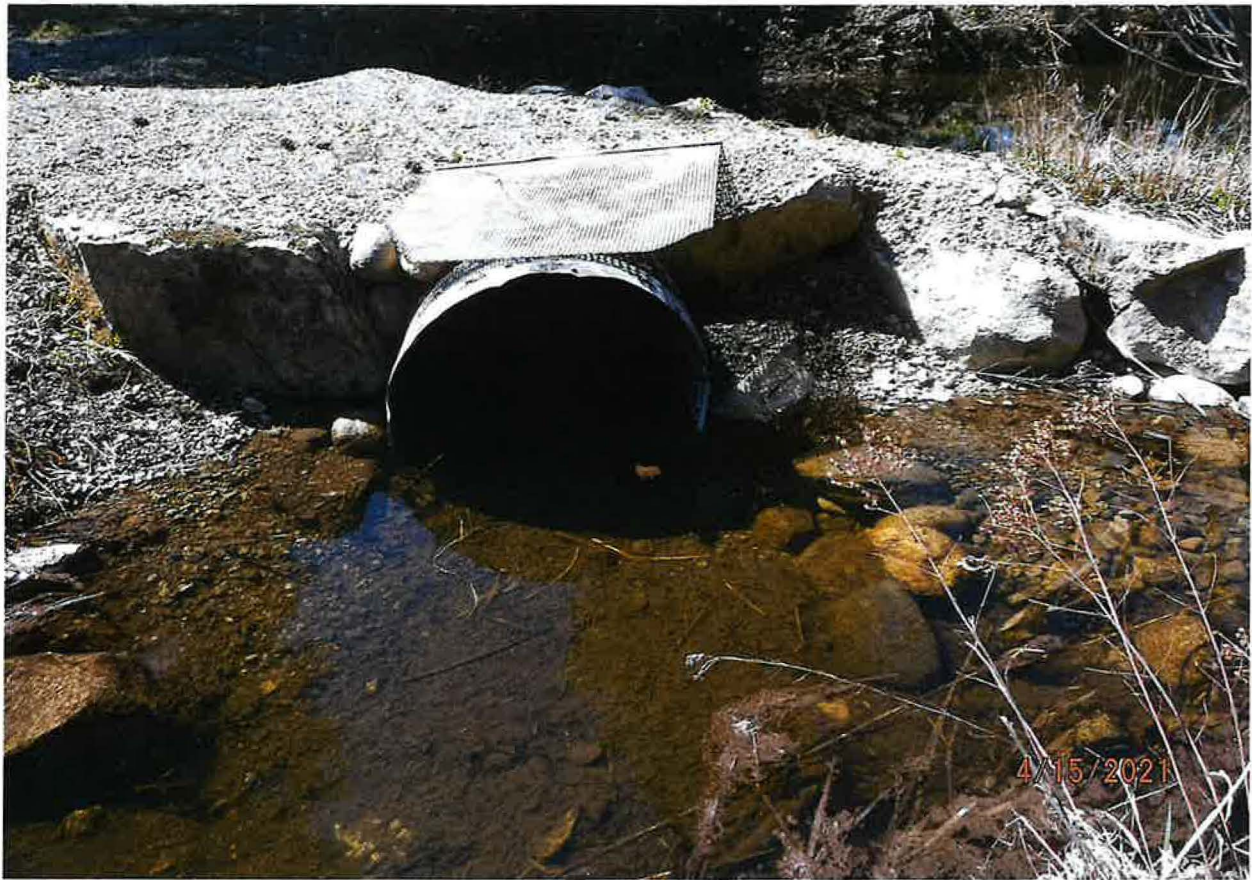
POD – 24 INCH CORRUGATED PIPE FROM CREEK – LOOKING TOWARD POND (4/15/2021)
