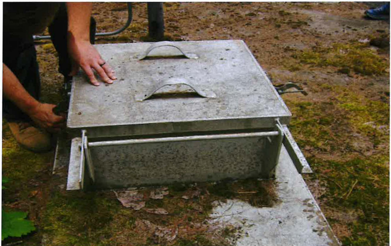
30,000 GALLON STORAGE TANK ACCESS HATCH
