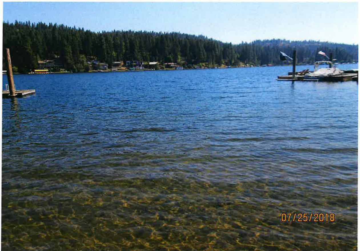
POD – 2EA SUBMERGED SCREENED INTAKE PIPES IN LAKE COEUR D'ALENE
