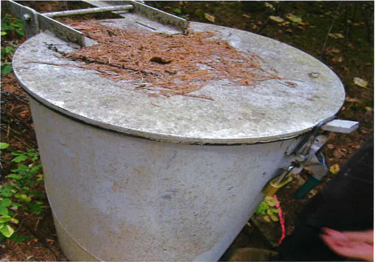
10,000 GALLON STORAGE TANK ACCESS HATCH
