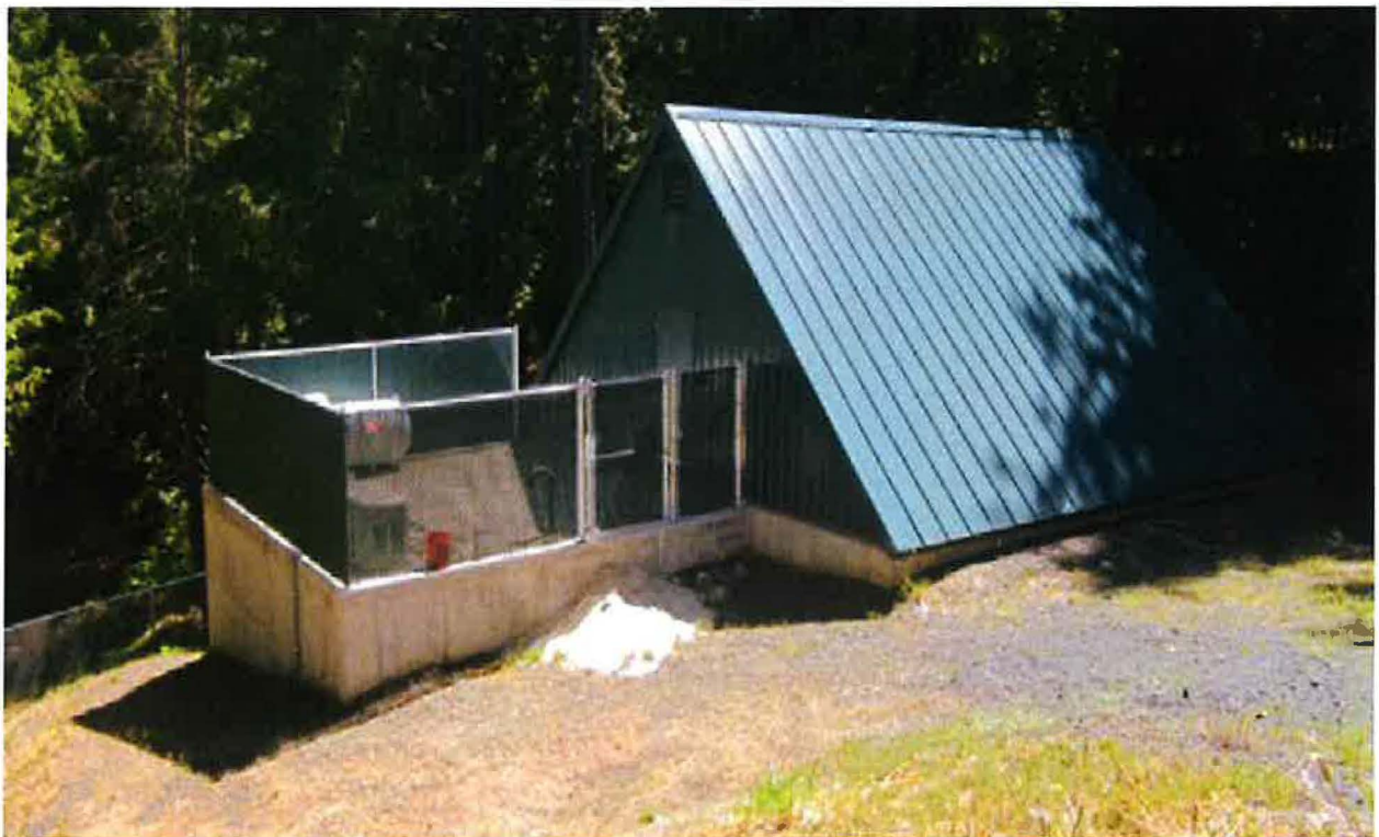
SLOW SAND FILTER BYA AND CONTACT CHAMBER
