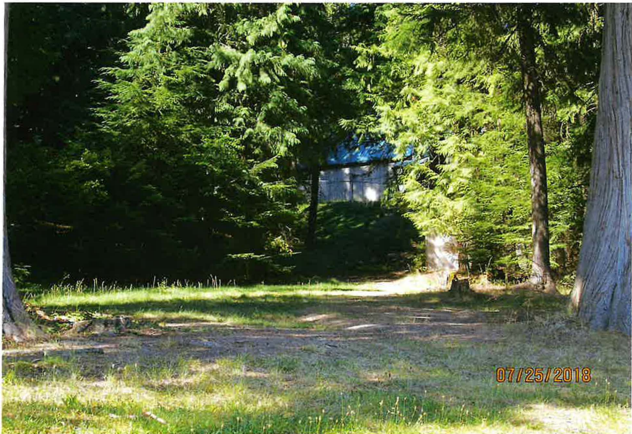
INTAKE PIPES FROM LAKE ROUTE TO PUMP STATION IN BACKGROUND OF PHOTOGRAPH
