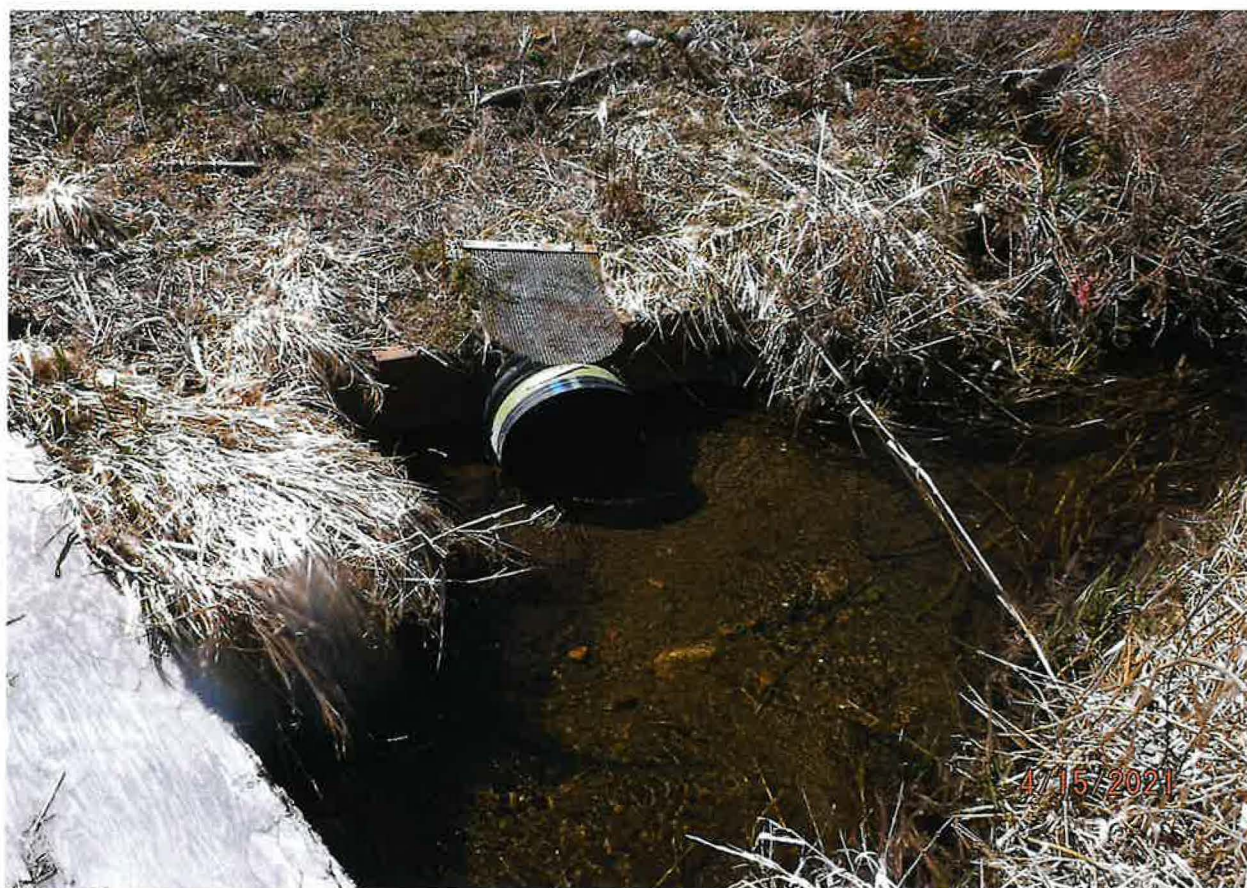
POD – INFLOW PIPE TO POND – PHOTO TAKEN 4/15/2021
