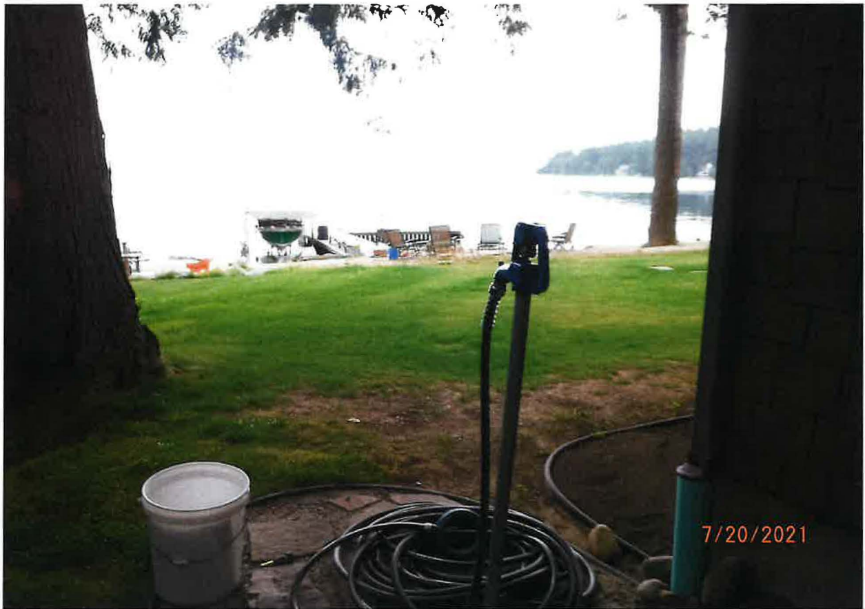
5 GAL BUCKET MEASUREMENTS TAKEN FROM FROST FREE HYDRANT
