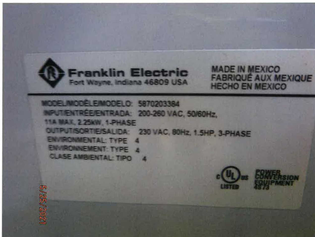
WELL D0055505 PUMP CONTROLLER – 1.5 HP PUMP INSTALLED IN WELL
