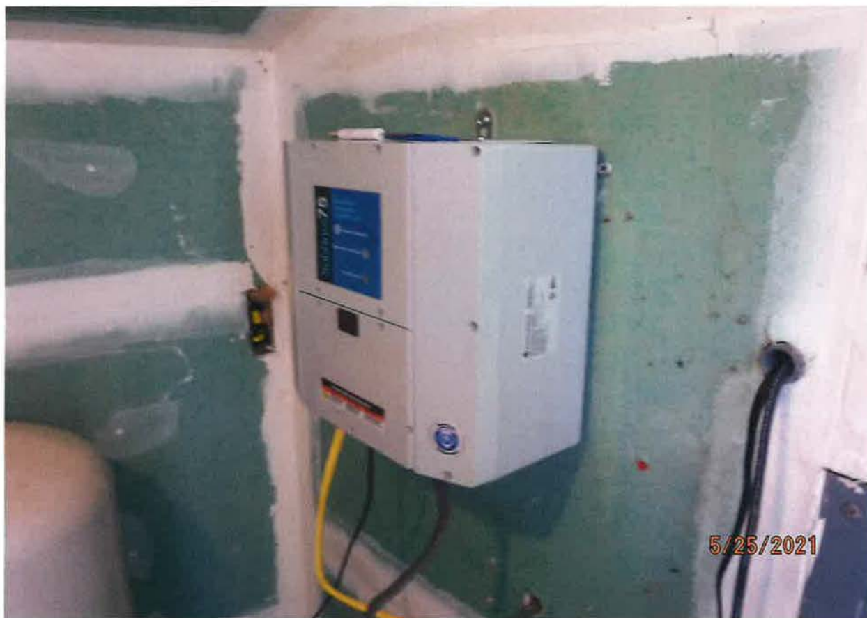
WELL D0055505 PUMP CONTROLLER – 1.5 HP PUMP INSTALLED IN WELL
