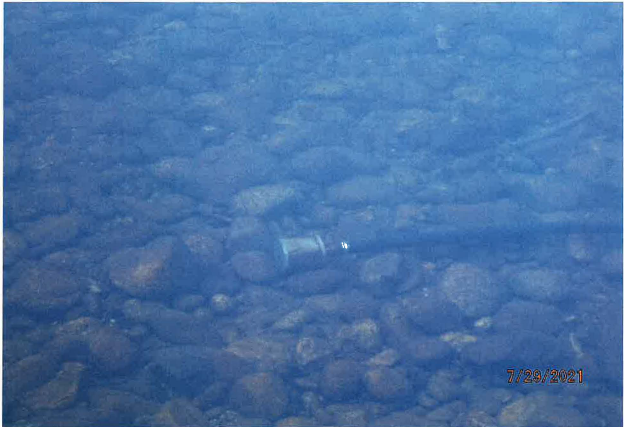
SCREENED INTAKE PIPE
