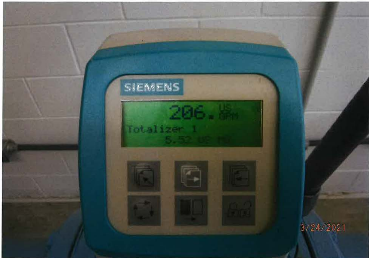
EAST WELL – FLOWMETER MEASUREMENT 206 GPM
