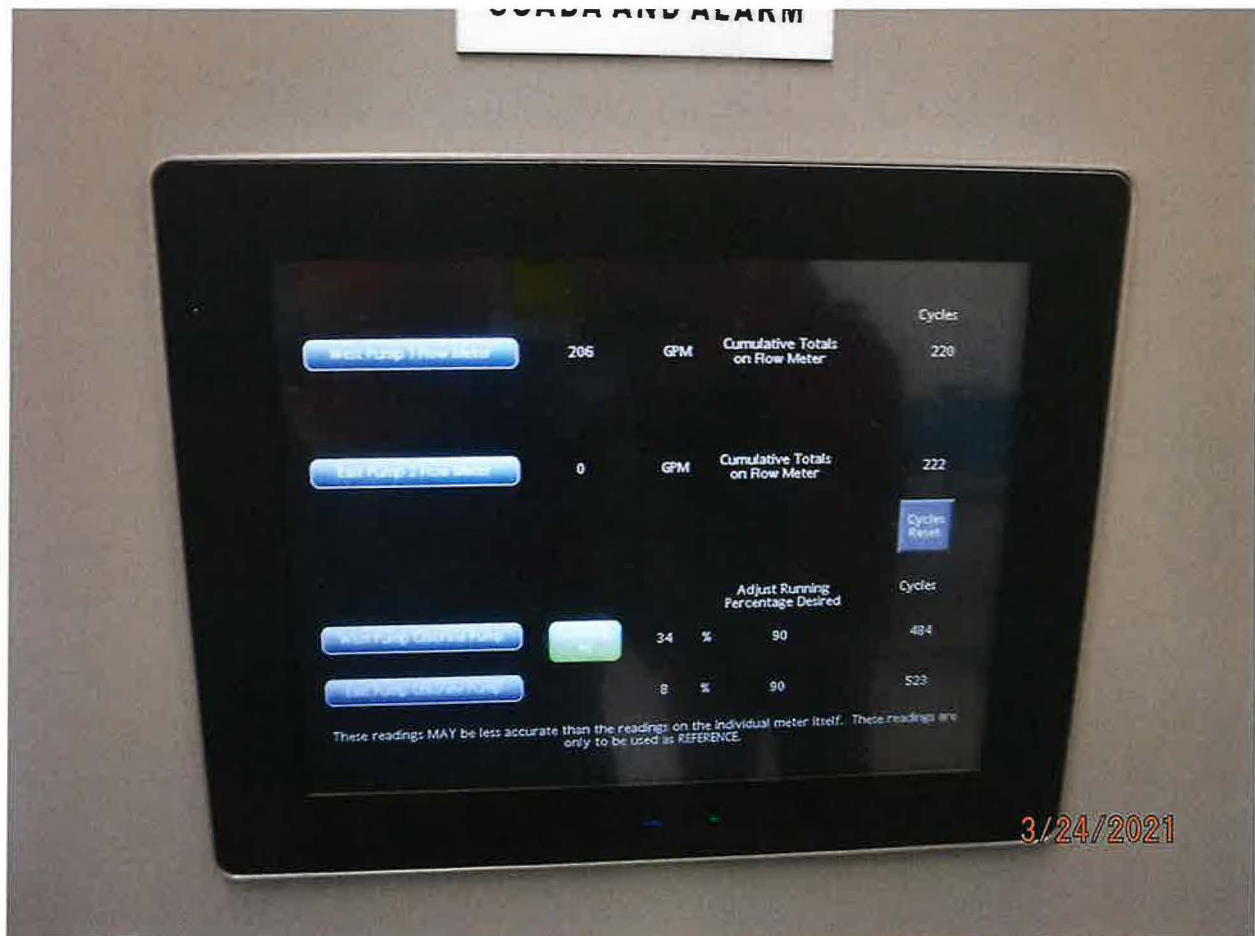
WATER SYSTEM SCADA CONTROL PANEL
