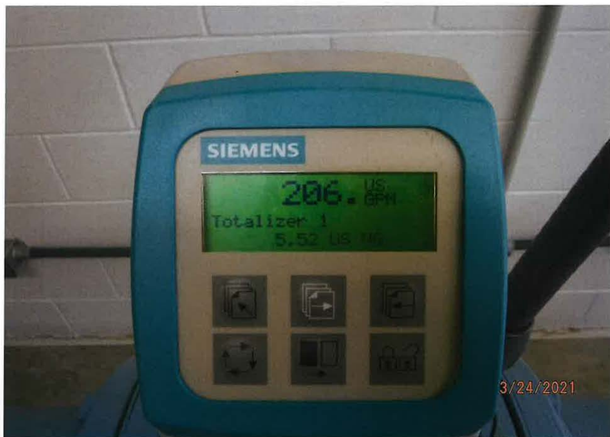
WEST WELL – FLOWMETER MEASUREMENT 206 GPM
