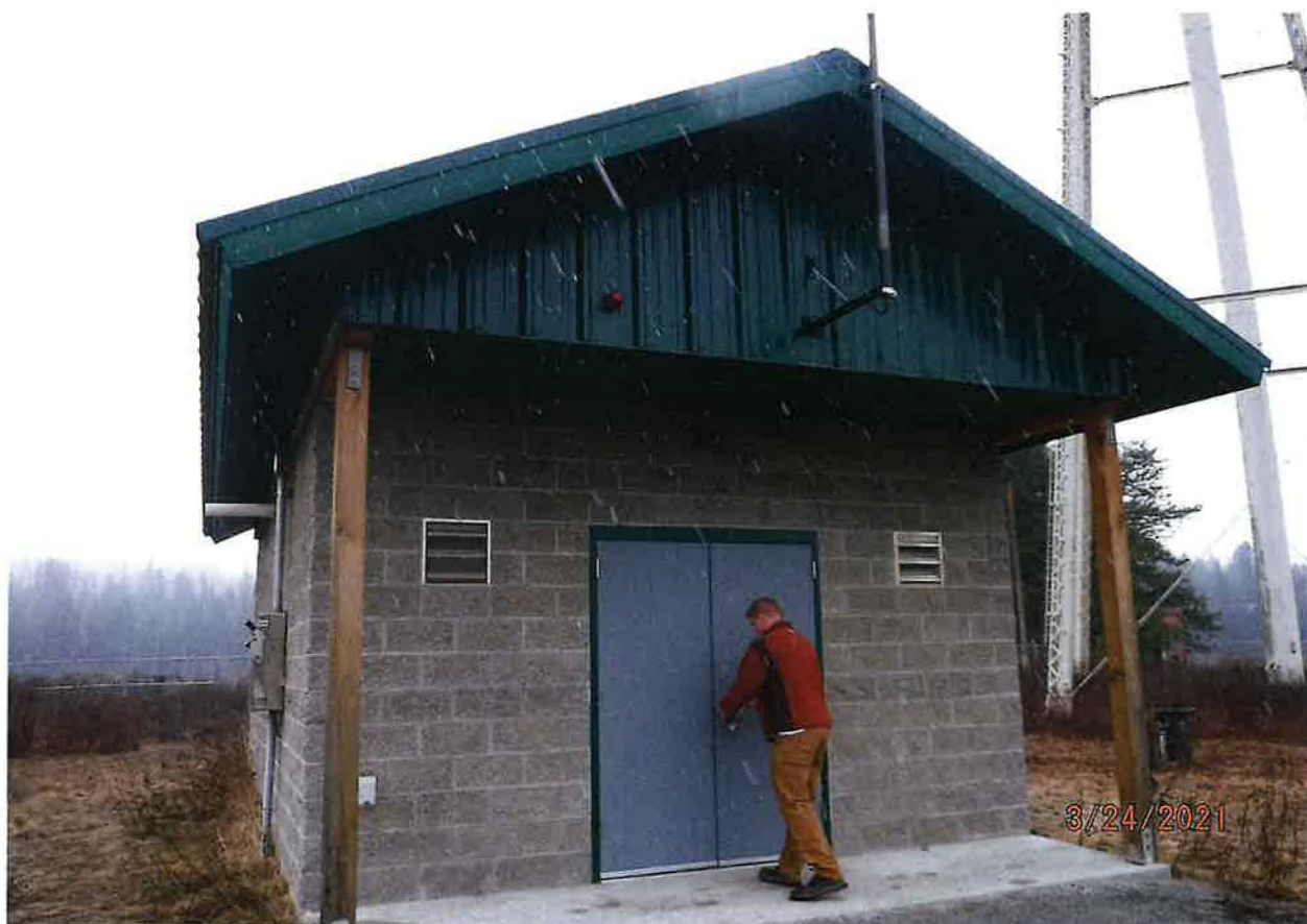
DIVERSION WORKS PUMP HOUSE
