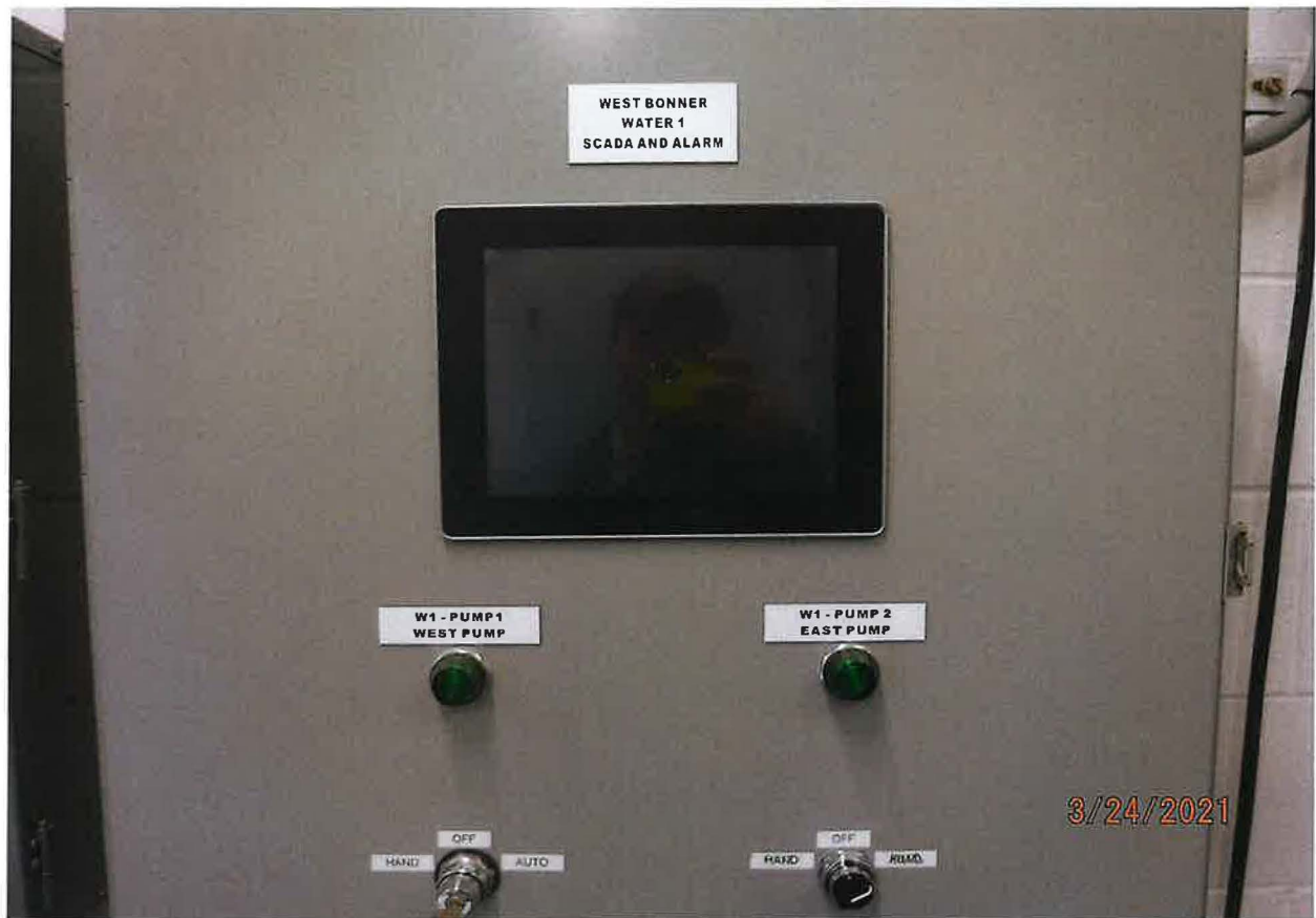
WATER SYSTEM SCADA CONTROL PANEL
