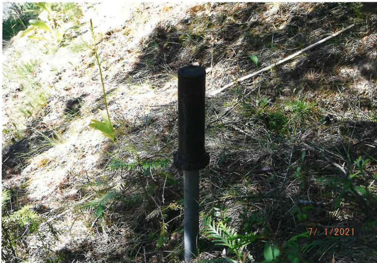
RAINBIRD SPRINKLERS INSTALLED AT INTERVALS ON BOTH SIDES OF ROADWAY TO IRRIGATE
