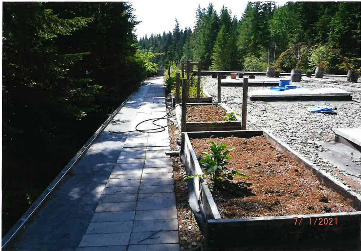
IRRIGATION OCCURING ON ROOF OF HANGER BY SOAKER HOSE
