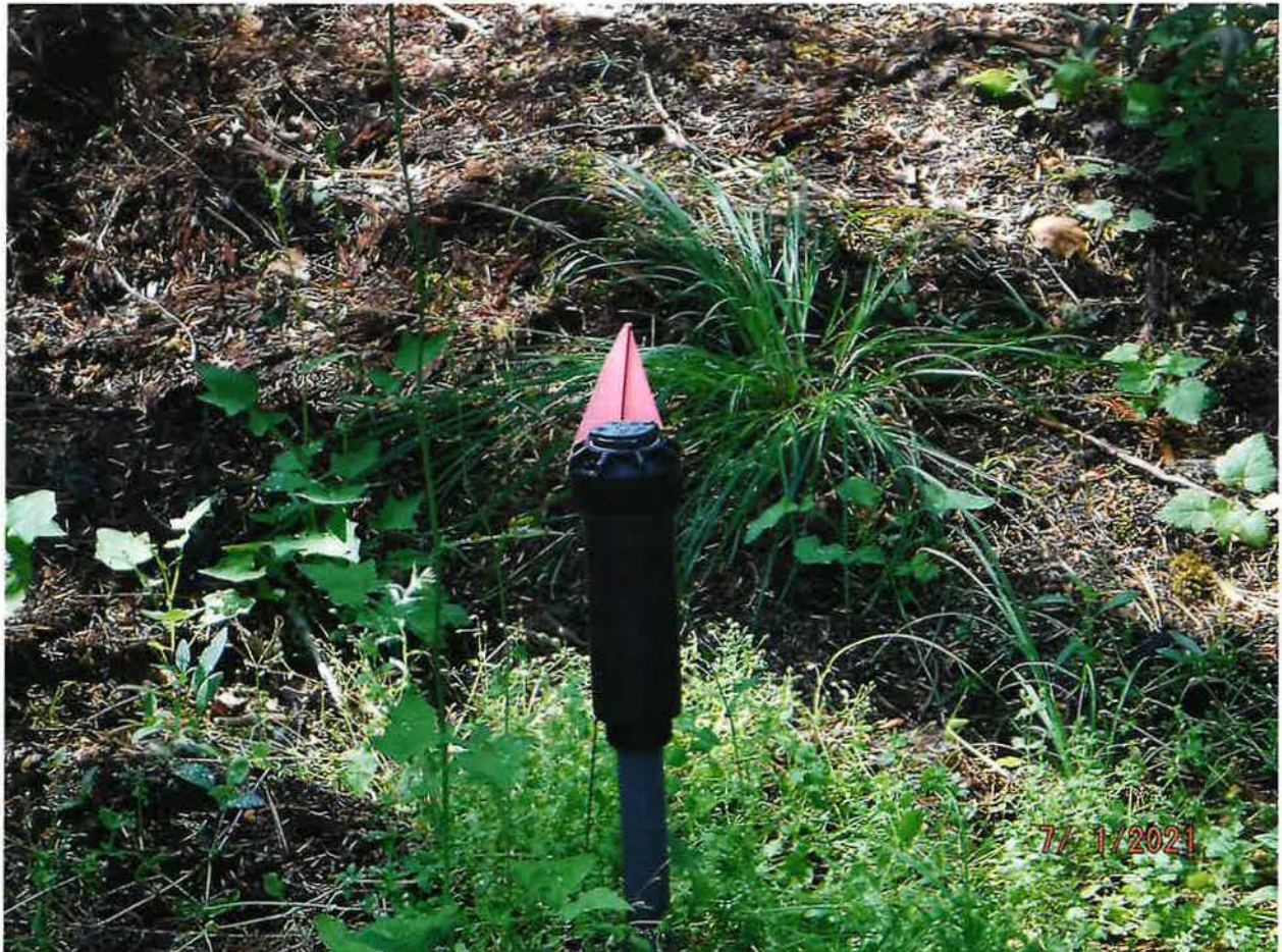
IRRIGATION/IRRIGATION FROM STORAGE POU – EXAMPLE RAINBIRD SPRINKLERS USED IN SYSTEM
