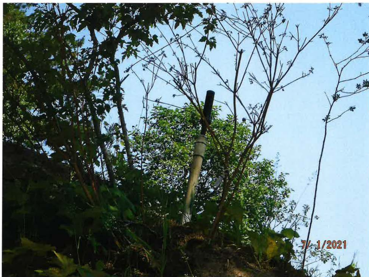
RAINBIRD SPRINKLERS INSTALLED AT INTERVALS ON BOTH SIDES OF ROADWAY TO IRRIGATE
