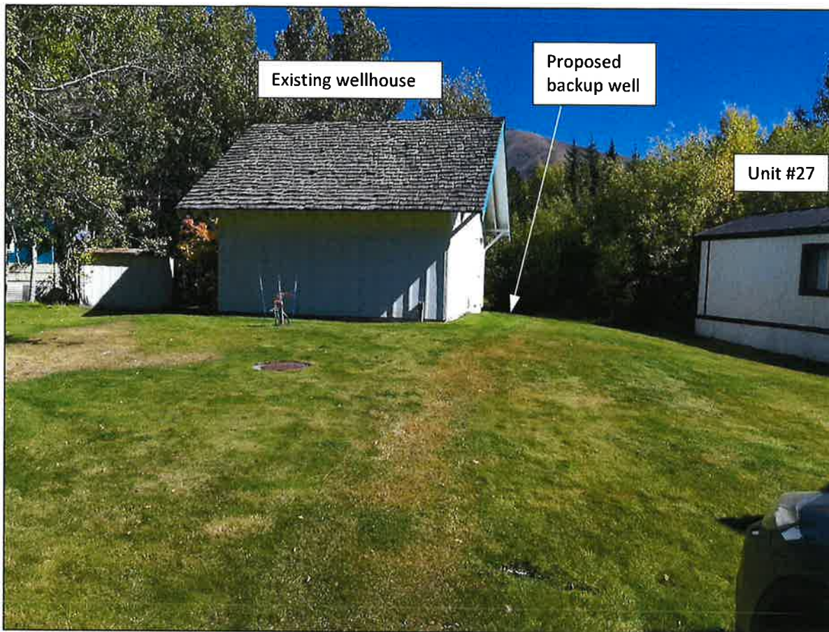
Water Right 37-8119. Photograph looking east toward the existing wellhouse on September 29, 2020.
