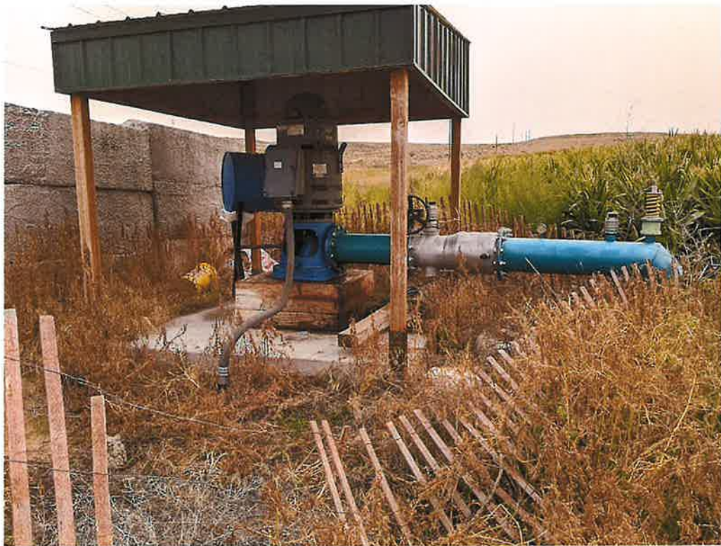
Well and Pump Installation
