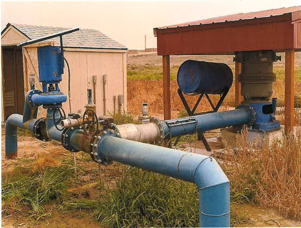
Pump and Well Installation
