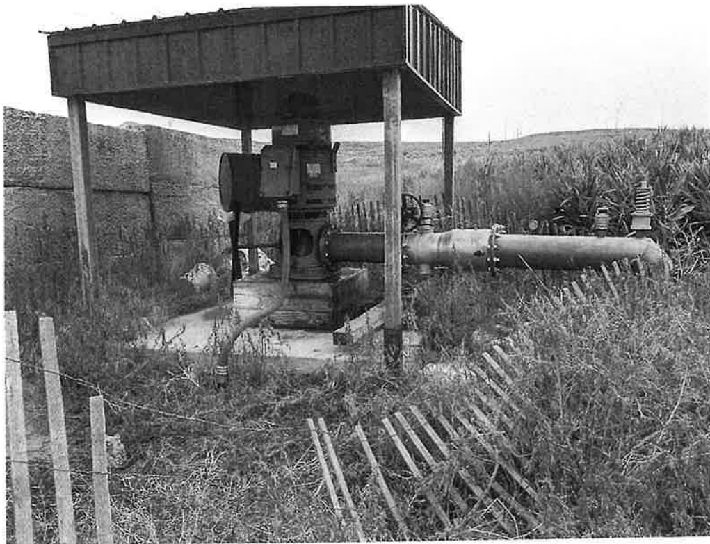
Well and Pump Installation
