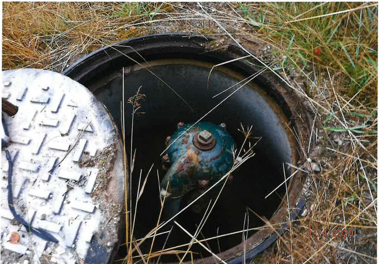
POD – WELL D0054541 LOCATED IN NE¼NW¼
