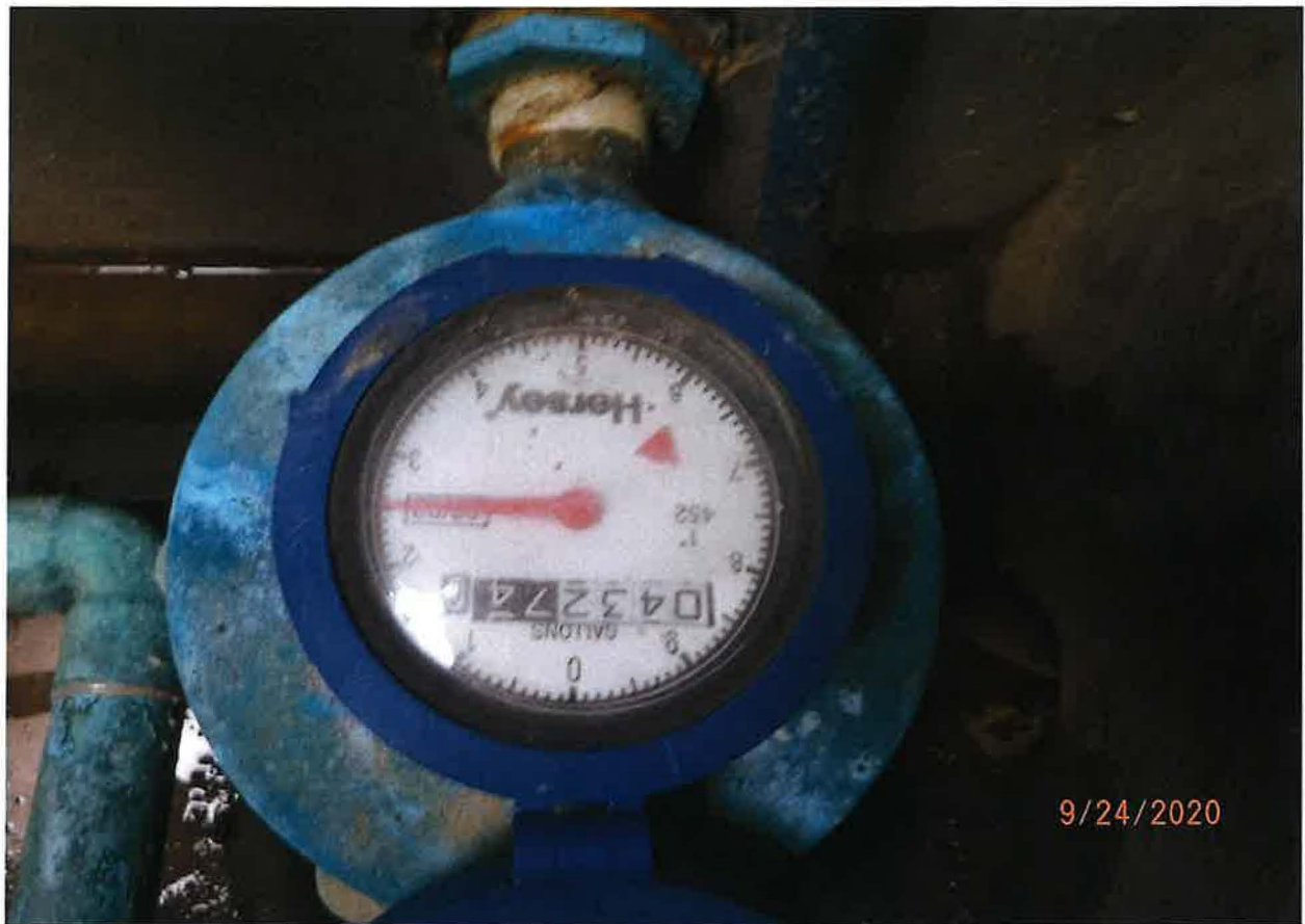
FLOWMETERS INSTALLED CAPTURING VOLUME DATA FROM 3,000 GALLON TANK TRANSFERRED TO 9,000 GALLON TANK PRIOR TO SYSTEM USE.
