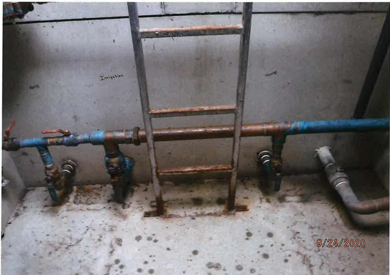
VAULTED 9,000 GALLON STORAGE RESERVOIR WATER WORKS
