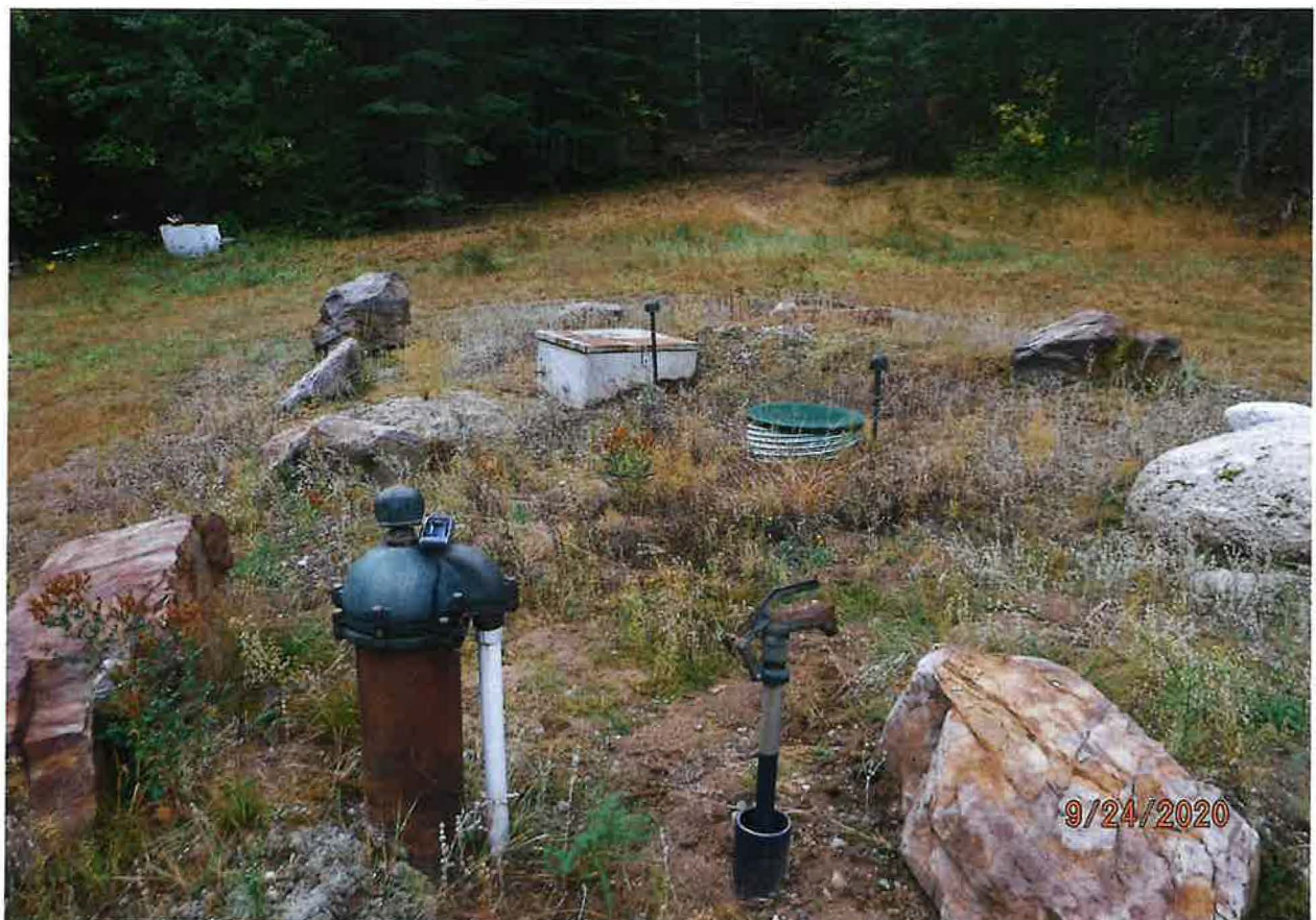
3,000 GAL STORAGE TANK LOCATED IN NE¼NW¼
