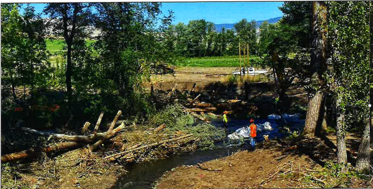
Figure 3-8. Construction of an apex log jam to bifurcate flows into restored side channel.
