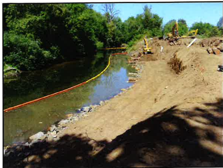
EXAMPLE OF FLOATING SILT CURTAIN PLACEMENT
