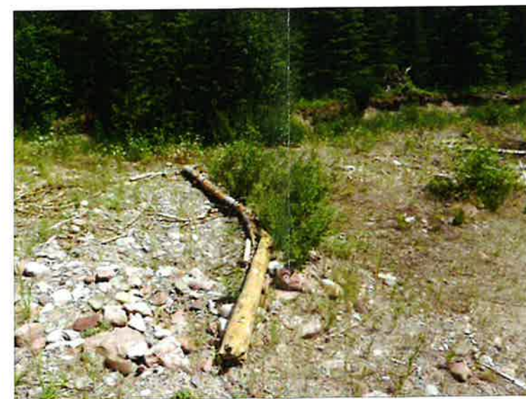
EXAMPLE OF A CONSTRUCTED VEGETATED BRUSH TRENCH
