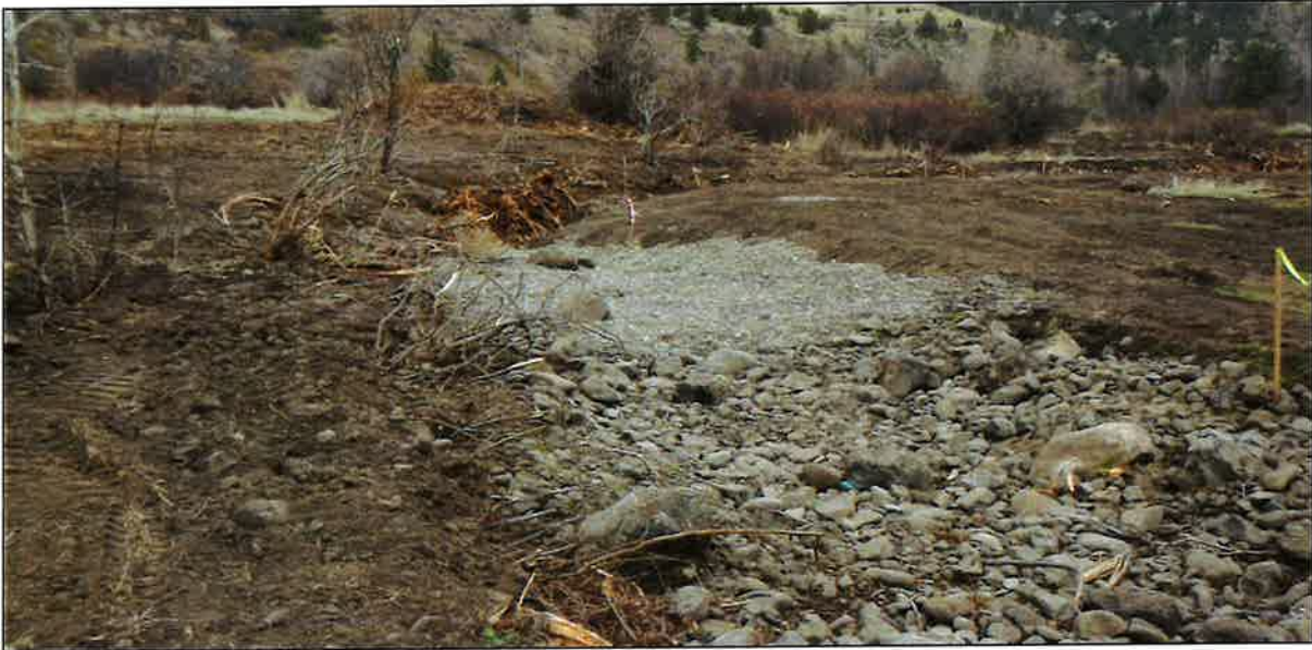
Figure 3-7. Construction of a riffle that transitions into a tailout and pool feature with a large wood bank structure.
