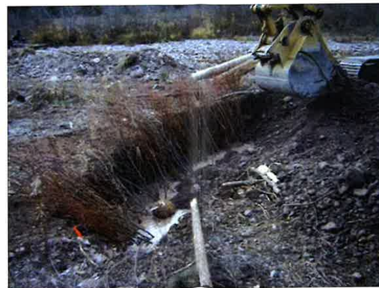
EXAMPLE OF A VEGETATED BRUSH TRENCH INSTALLATION
