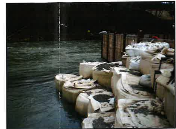
EXAMPLE OF BULK BAG PLACEMENT
