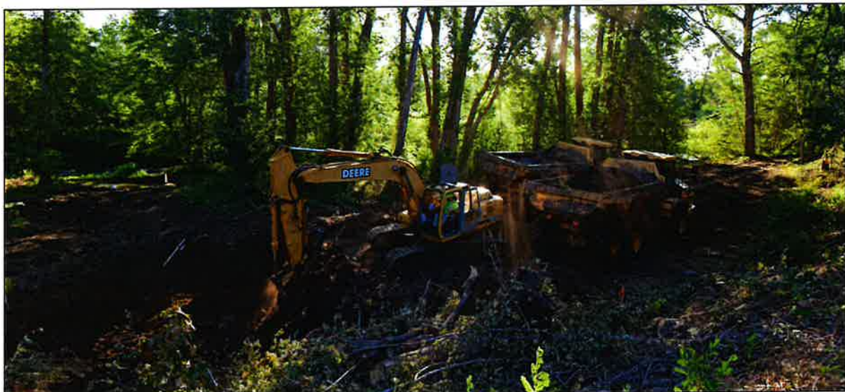
Figure 3-3. Example of selective excavation and removal of soil while maintaining existing trees.
