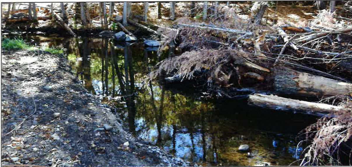
Figure 3-5. Large wood structure buried into bank for stability.
