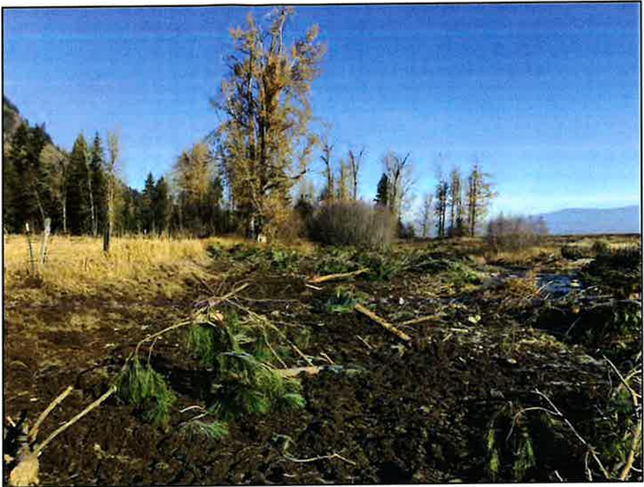
EXAMPLE OF CONSTRUCTED FLOODPLAIN ROUGHNESS ELEMENTS
